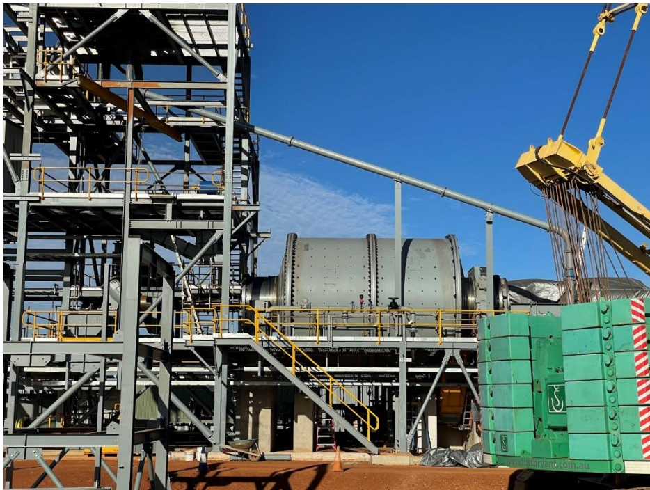
Figure 9 – Mill installation (photo 13 September).
