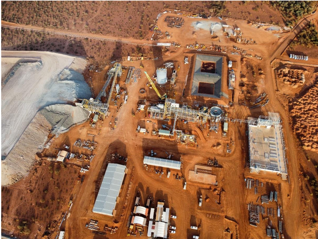
Figure 4 – Abra processing plant construction, workshops, and offices.
