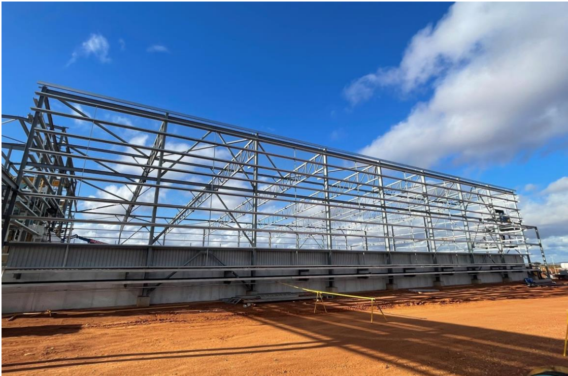
Figure 11 – Concentrate shed construction.
