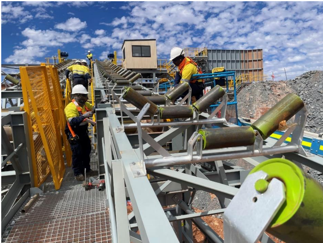
Figure 7 – Abra crushing section conveyor alignment work.
