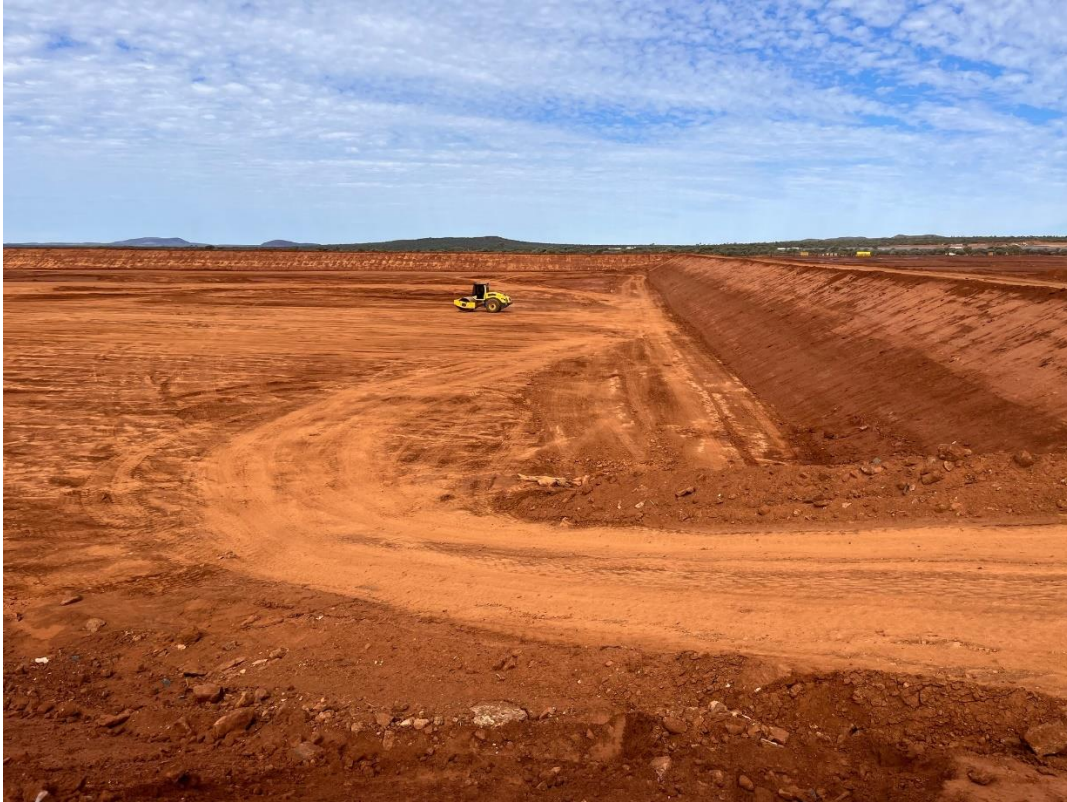
Figure 6 – Abra TSF construction with preparation for liner installation (photo 9 September).
