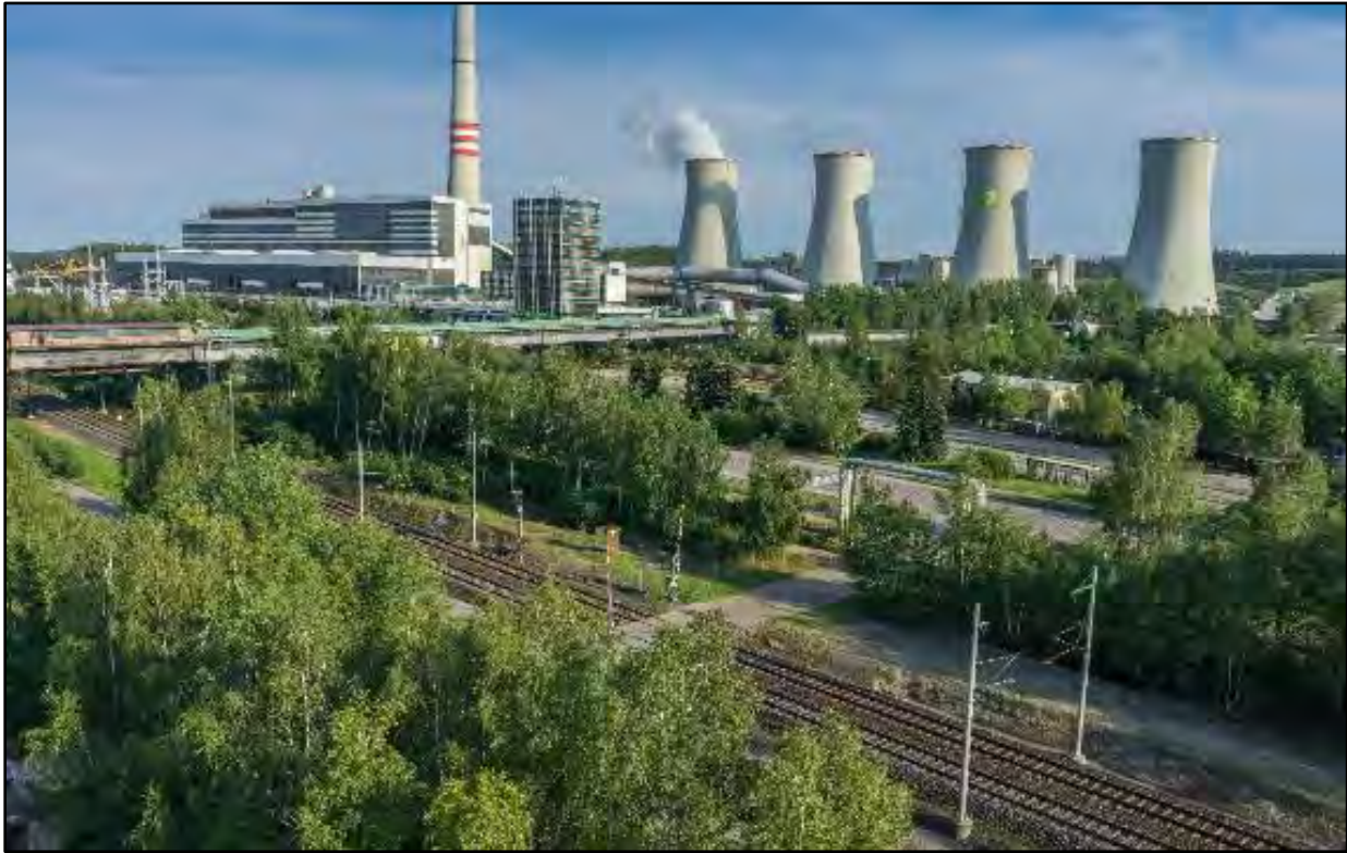
Figure 6-3: Current Power Plant
