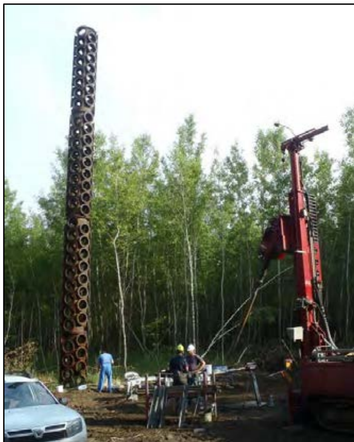
Figure 6-4: Historical Decantation Tower Located on Cell #3, Near Drill Holes T3-310, 311, and-318
