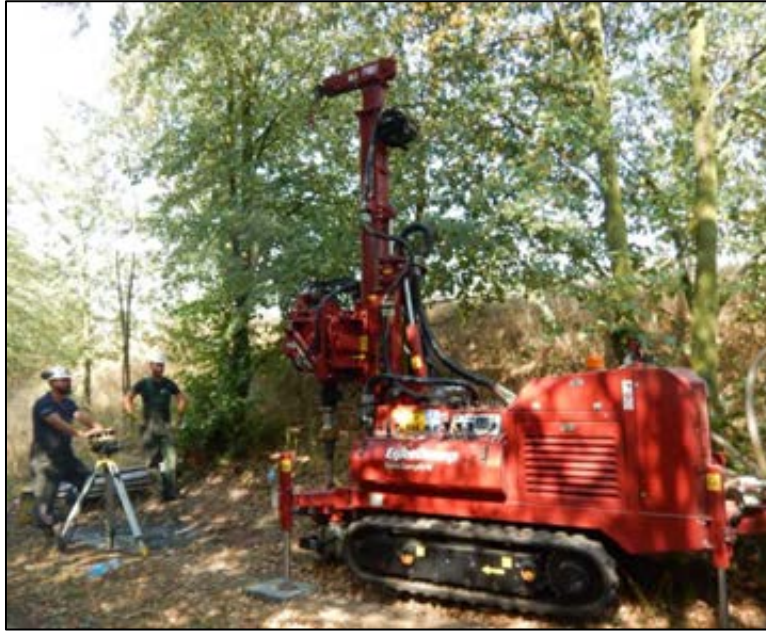
Figure 10-3: Eijkelkamp SonicSampDrill SRS Used for 2018 Sonic Drilling Investigation
