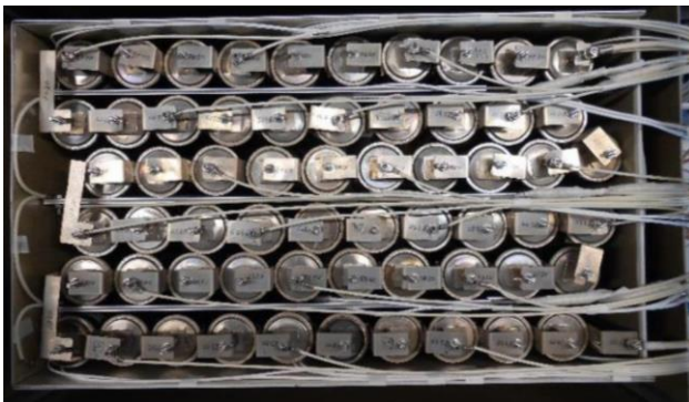
Figure 8 – Configuration of cells in battery module
