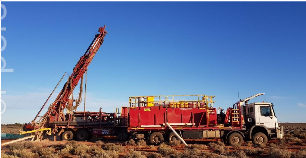
Figure 13: Drill rig on site at Glenloth Goldfield
