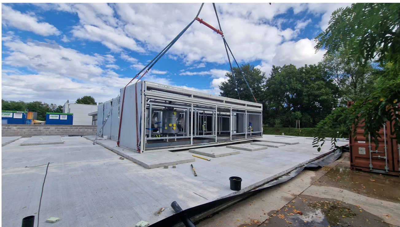
Positioning of the prefabricated containers at the Sorption-Demo Plant in Landau, Germany.
