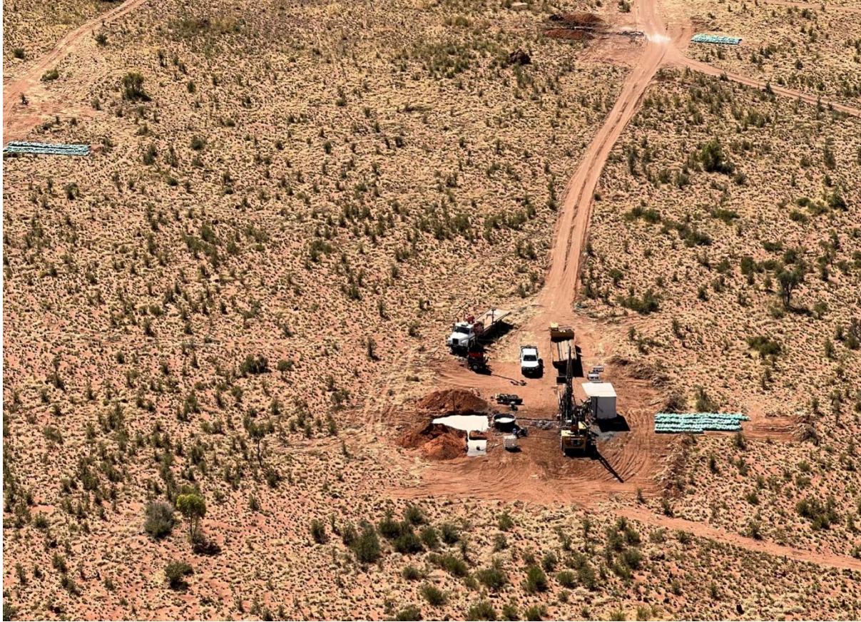
Figure 8-2: Drilling for geological and metallurgical samples
