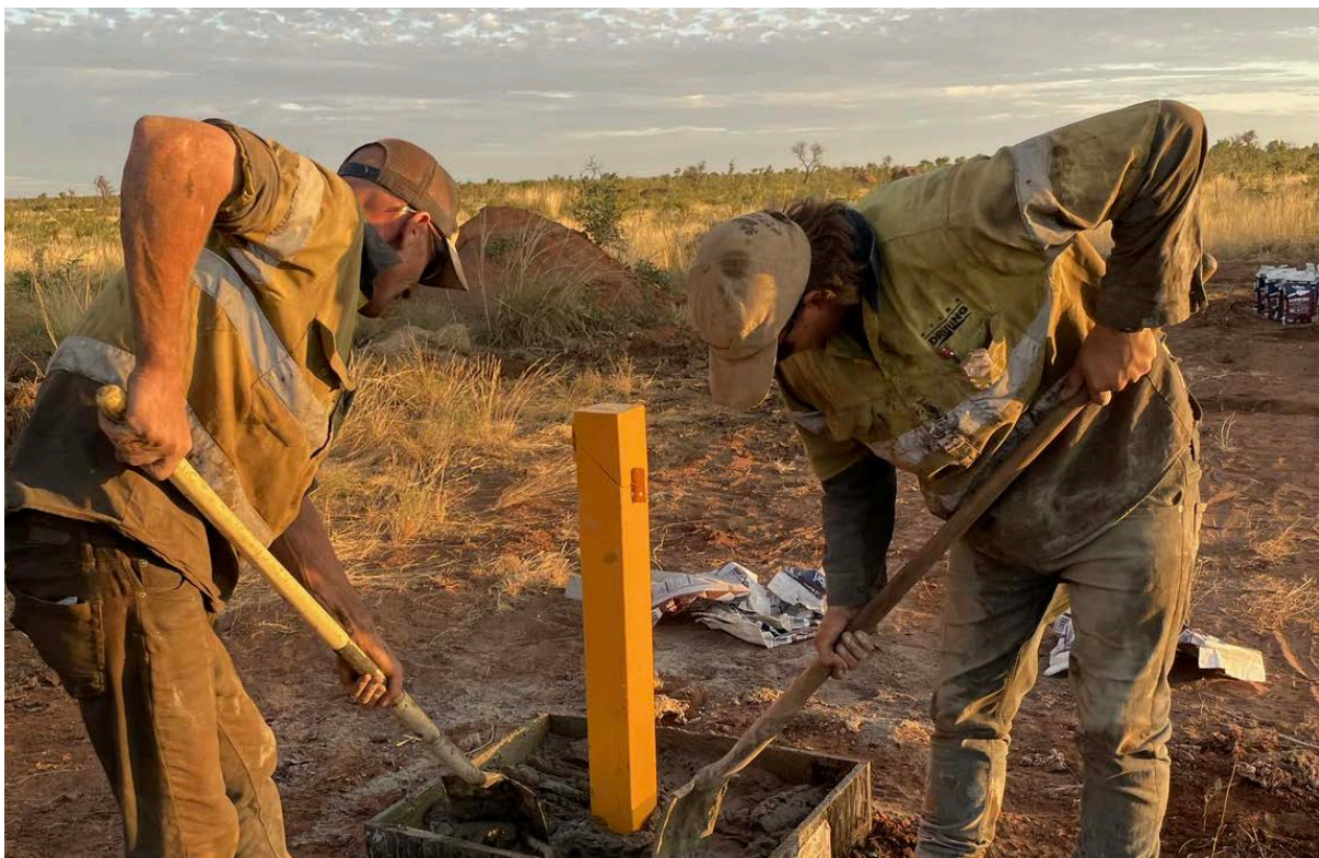
Figure 14-1: Water monitoring bore installation
