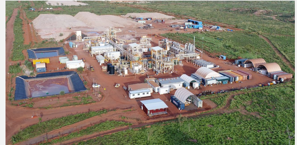
Northern Minerals Limited Browns Range Pilot Plant
