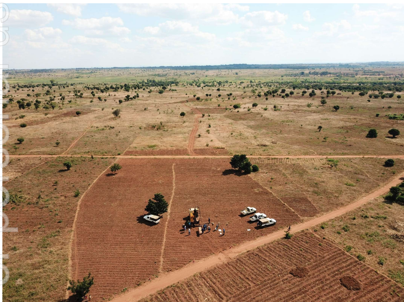
Figure 2: THR001 air-core drilling rig in operation at Kasiya, showing drill pads lightly cleared in the background
