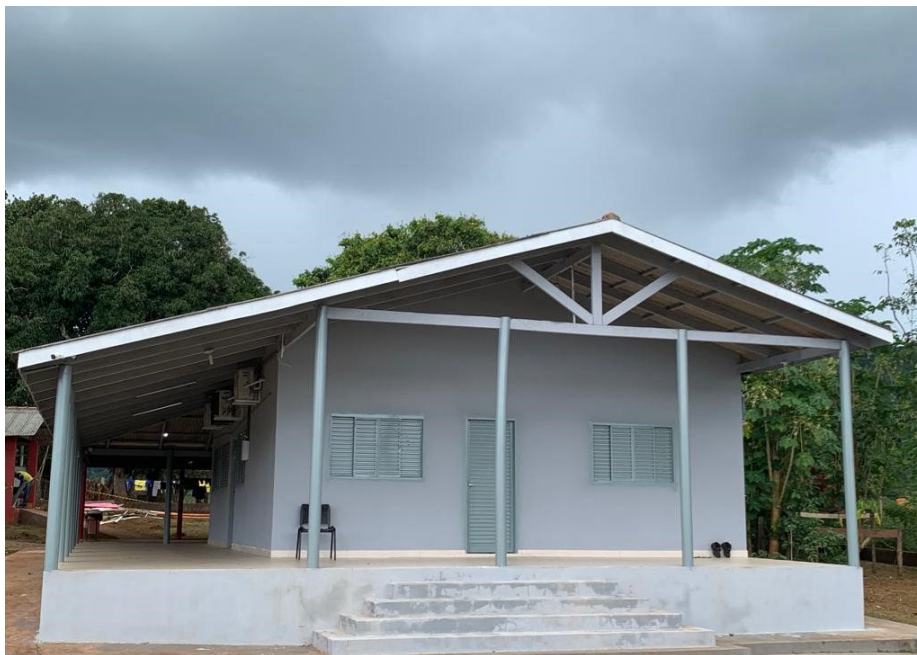
Figure 6: New On-site Accommodation at Jaguar
