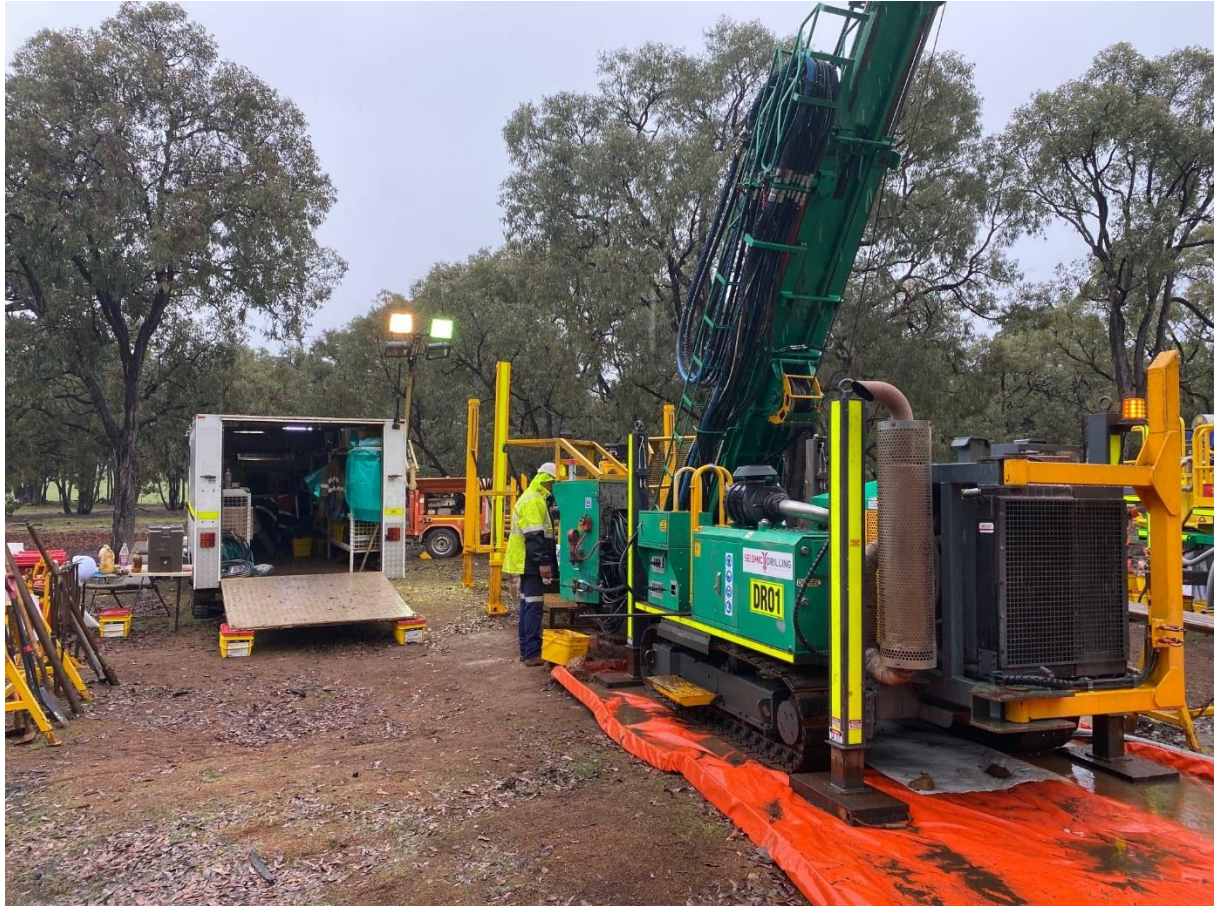
Photo 1: Diamond drilling at Coates Ni-Cu-PGE Project near Julimar.
