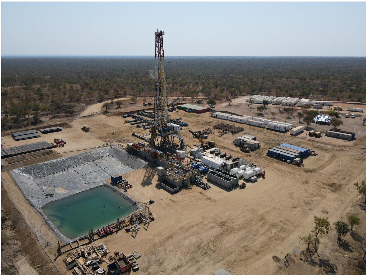
Figure 3 - Exalo Rig 202 at Mukuyu-1 wellsite preparing to commence drilling early September
