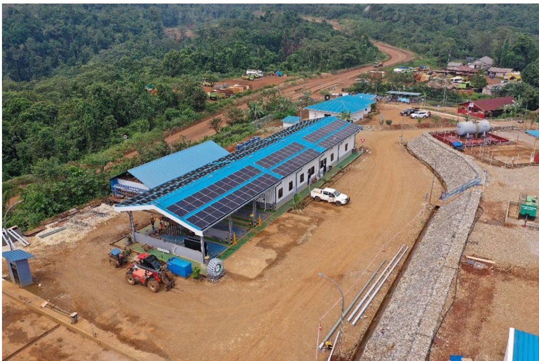
The existing 396kWp plus 250kWh battery storage project at the Hengjaya Mine
