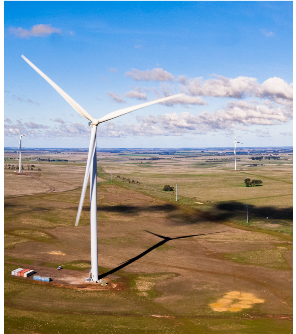
▲ Stockyard Hill Wind Farm
