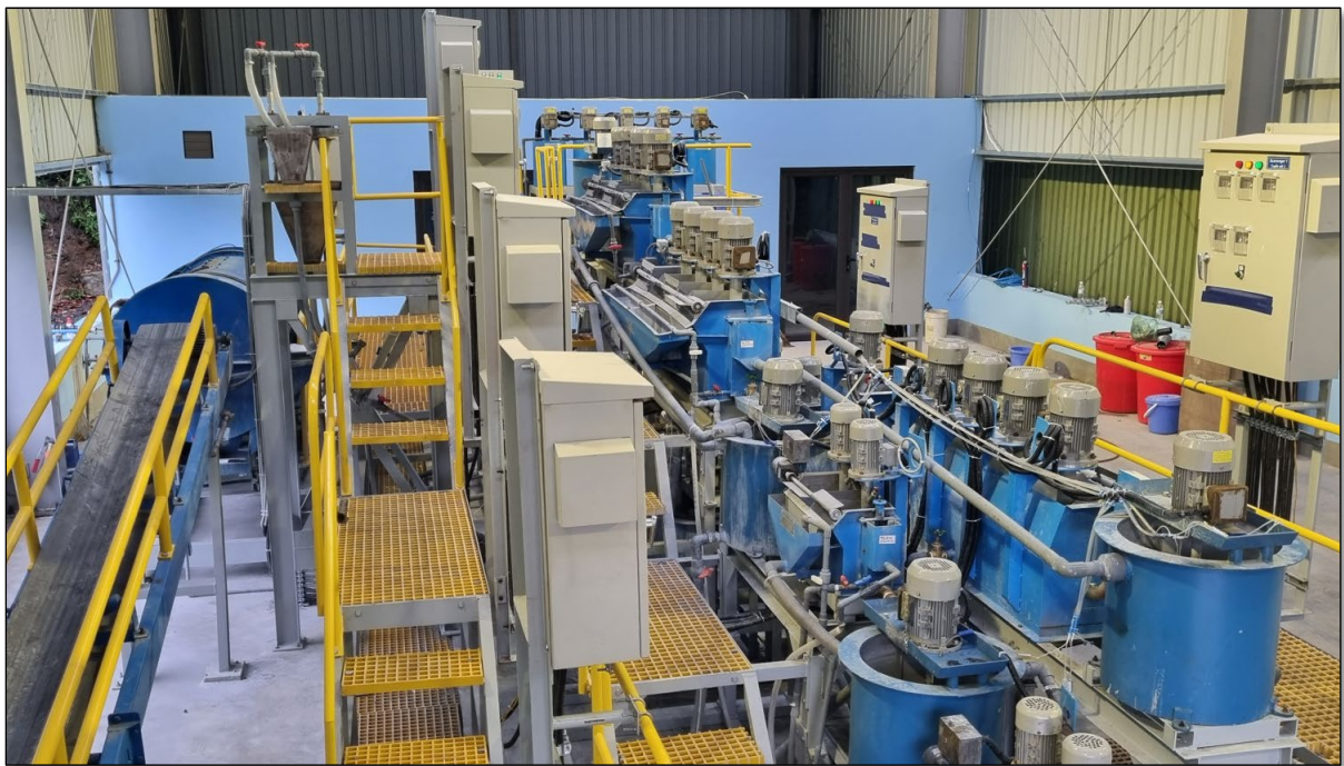
Figure 3: TKN Pilot Plant located at the mine site
