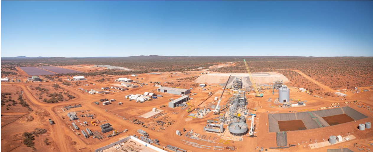
Figure 5 – Abra processing plant construction, power station, solar and administration buildings.
