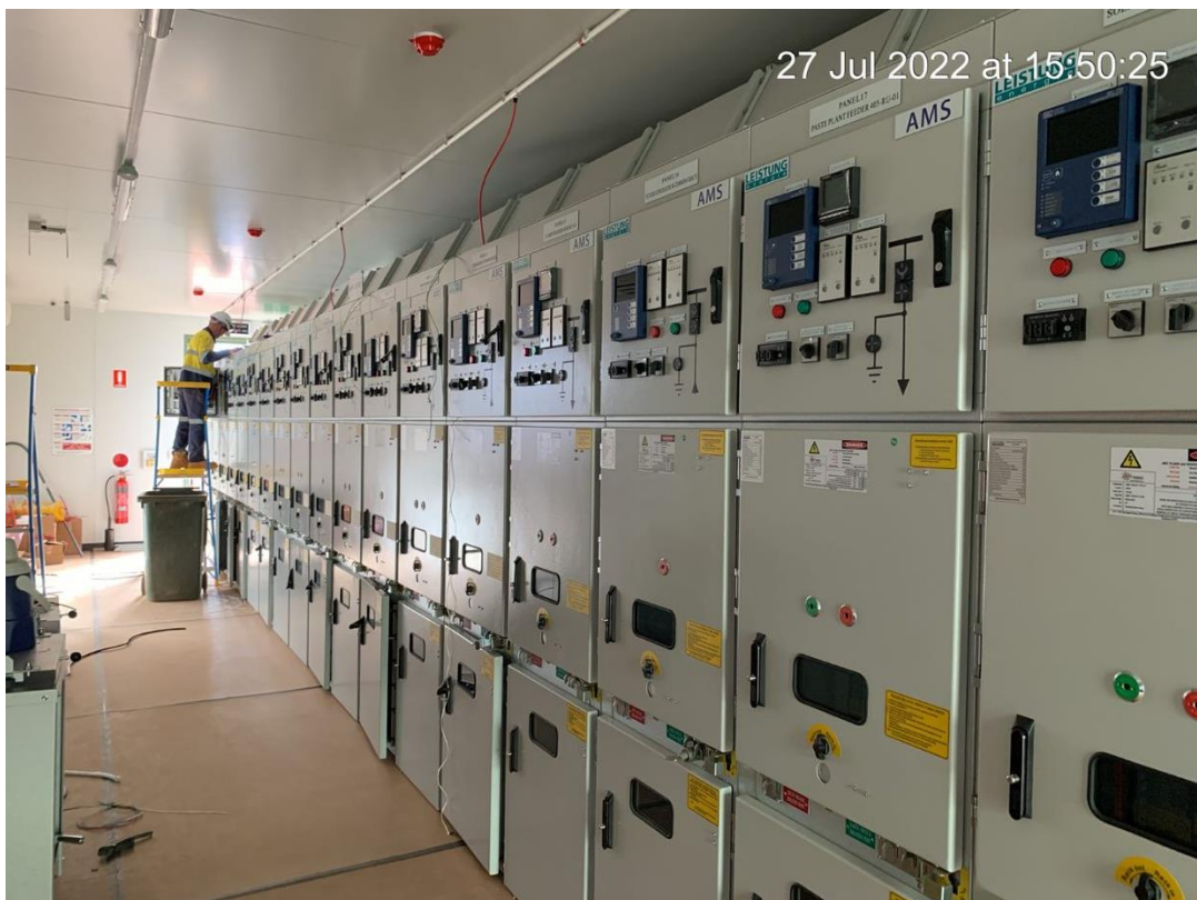
Figure 14 – Power station switch room (Pacific Energy).
