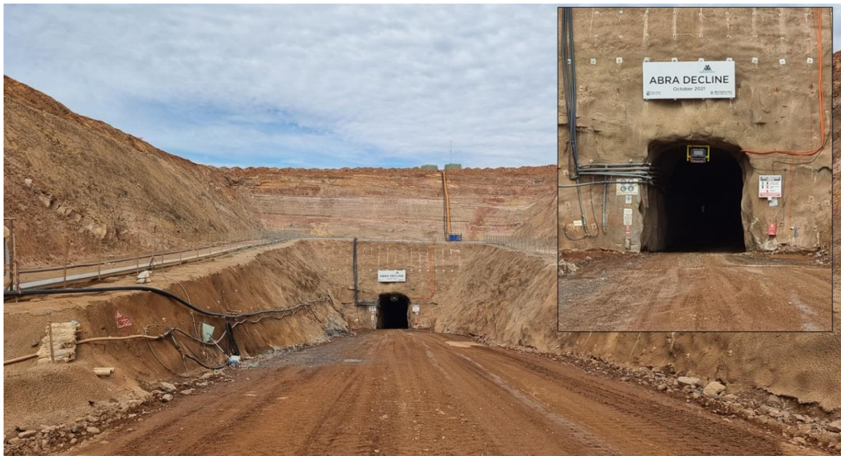
Figure 16 – Abra Box-cut and portal.
