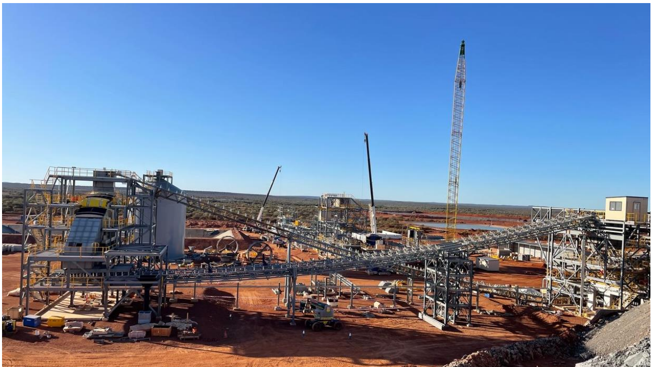
Figure 6 – Abra crushing & screening sections steel erection (photo: 12 August).
