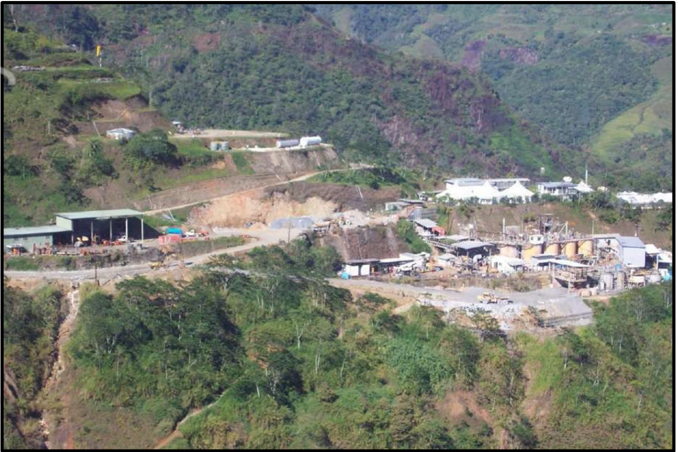
Figure 03: Aerial view of the mine and infrastructure
