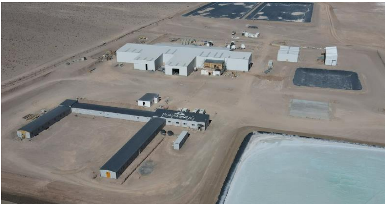
Figure 1. Rincon Lithium Project – 2,000tpa Operation Site Works
