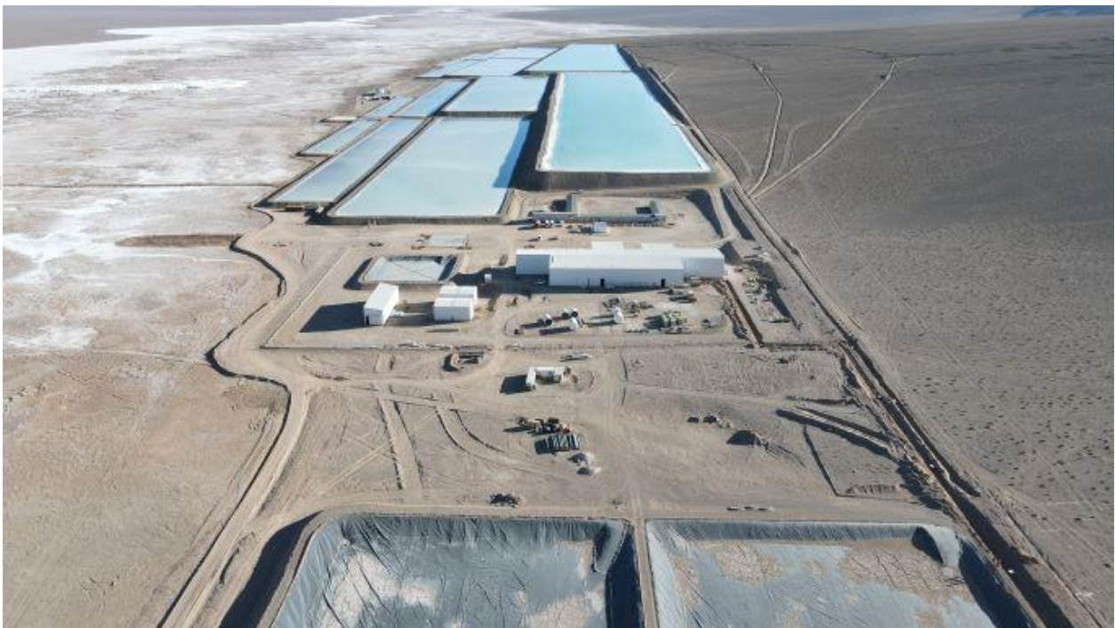
Figure 6. Rincon Lithium Project – 2,000tpa Operation Site Works
