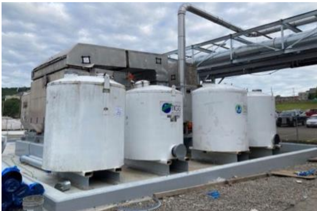
Figure 3: Condenser system with carbon to capture solvent
