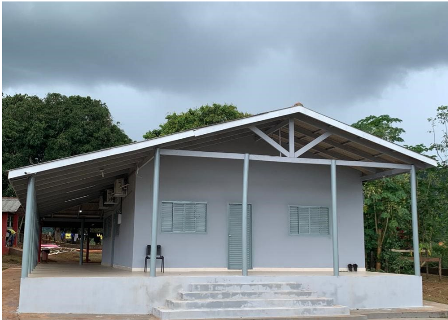
Figure 9 – New On-site Accommodation at Jaguar
