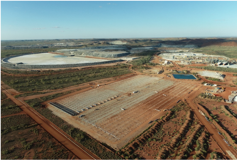
Above: Aerial view of 6MW solar farm under construction.
