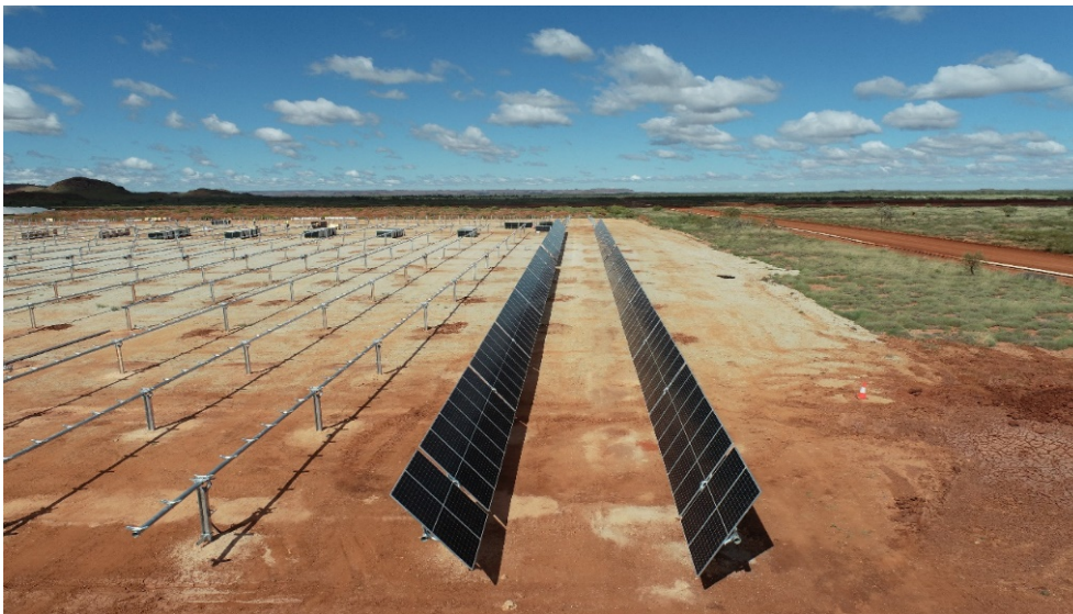
Above: 6MW solar farm under construction.
