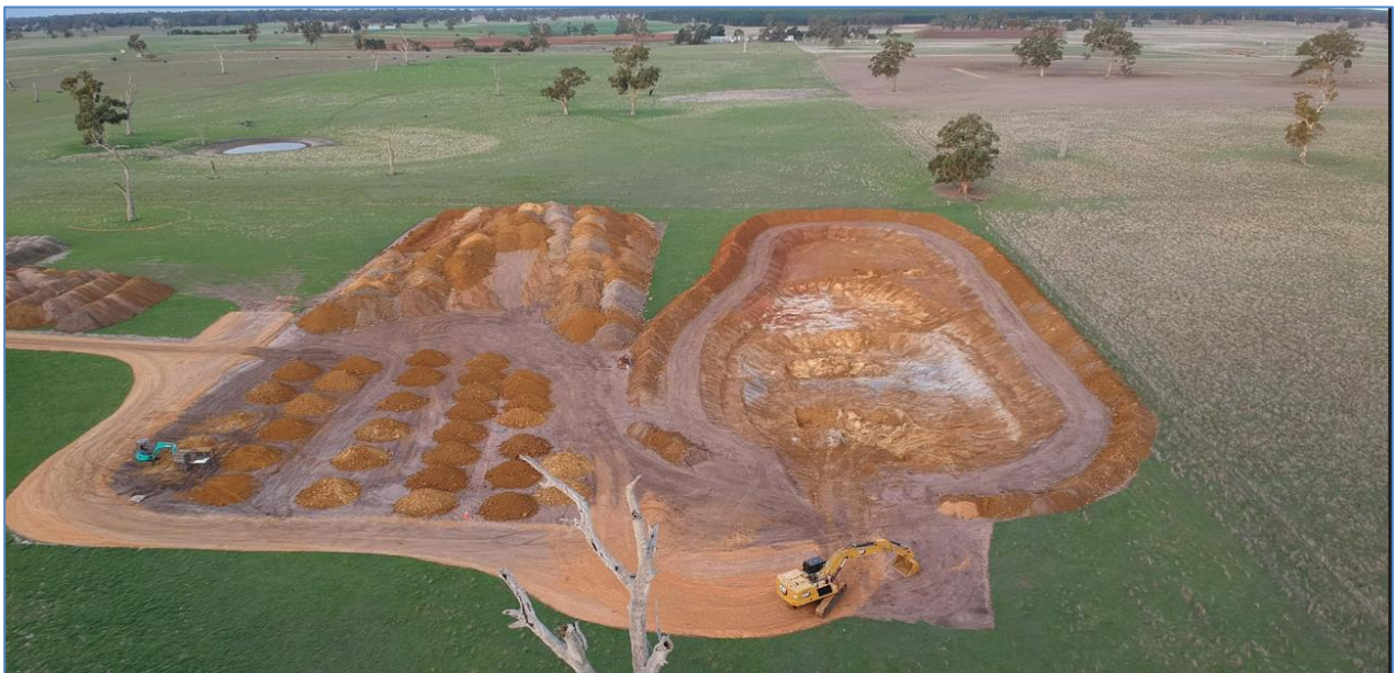
Trial mine at maximum excavation extents – 17 May 2022
