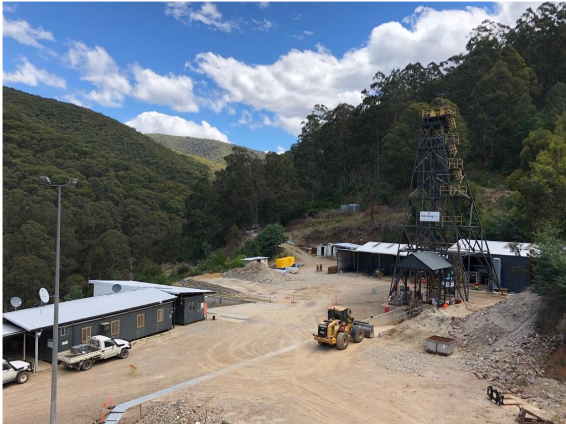
Figure 5: The Morning Star Gold Mine headframe and offices.
