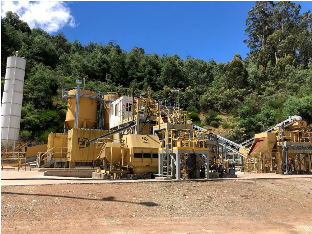
Figure 4: Gold processing plant at White Rock's Morning Star Gold Mine, NE Victoria
