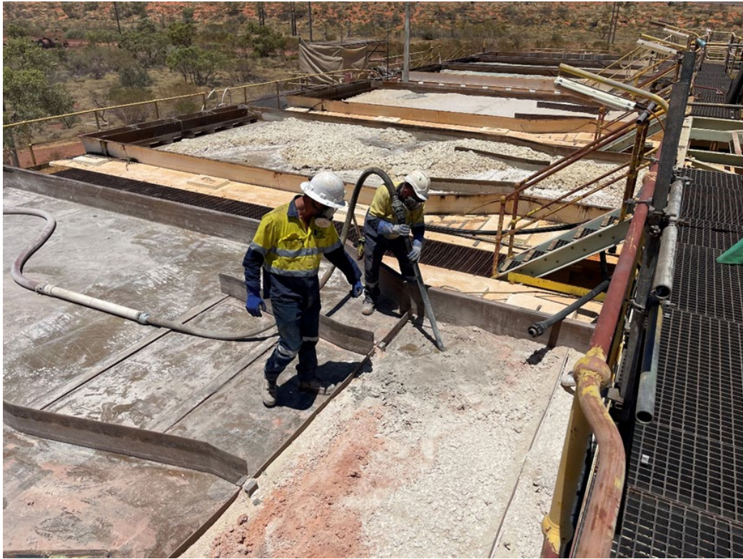
Image 2 / SX Mixer Settler clean-up top level
