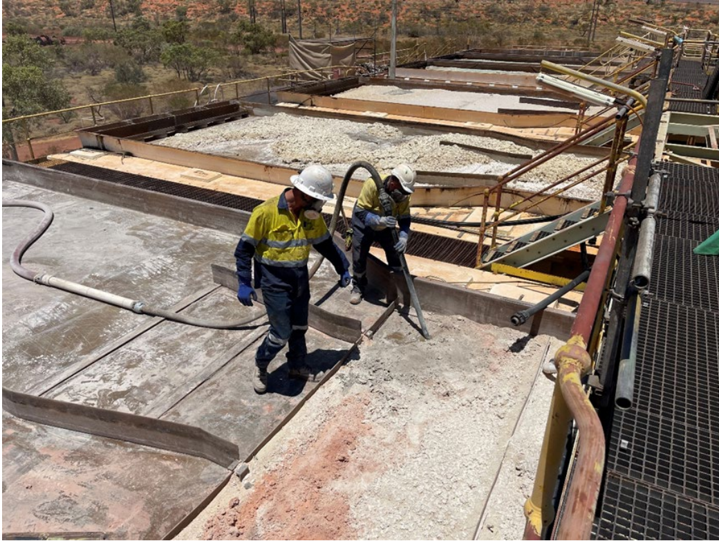
Image 2 / SX Mixer Settler clean-up top level
