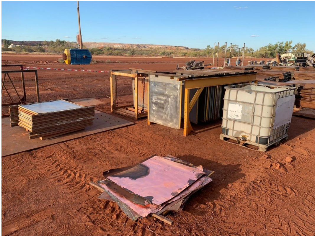
Image 5 / Removal of Cathodes
