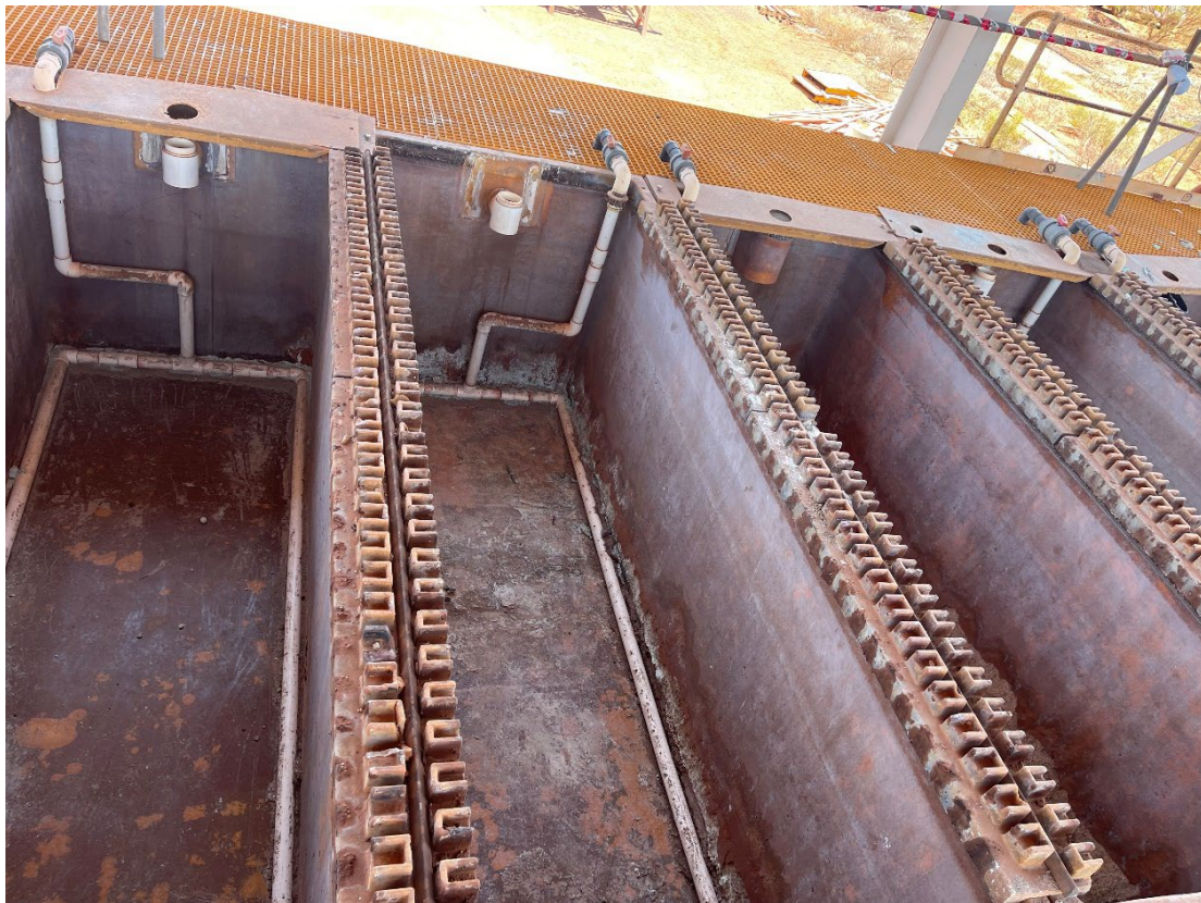
Image 9 / Cleaned EW Cells ready for condition inspection
