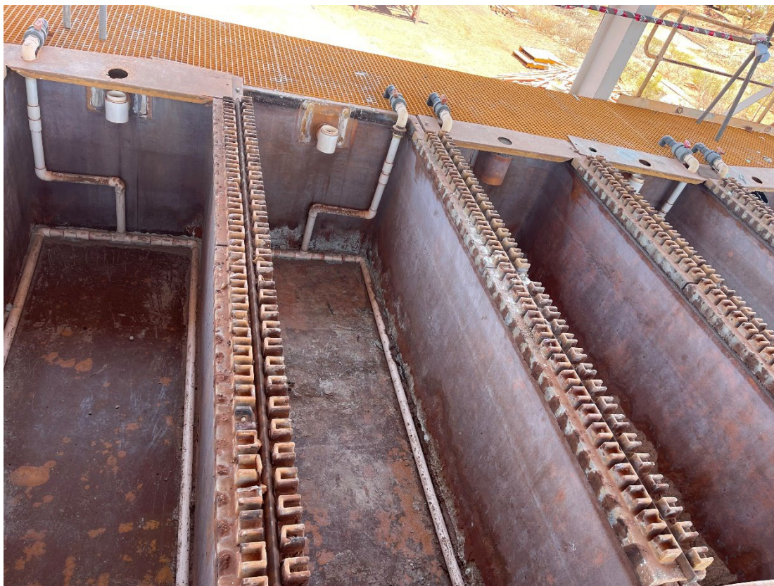
Image 9 / Cleaned EW Cells ready for condition inspection
