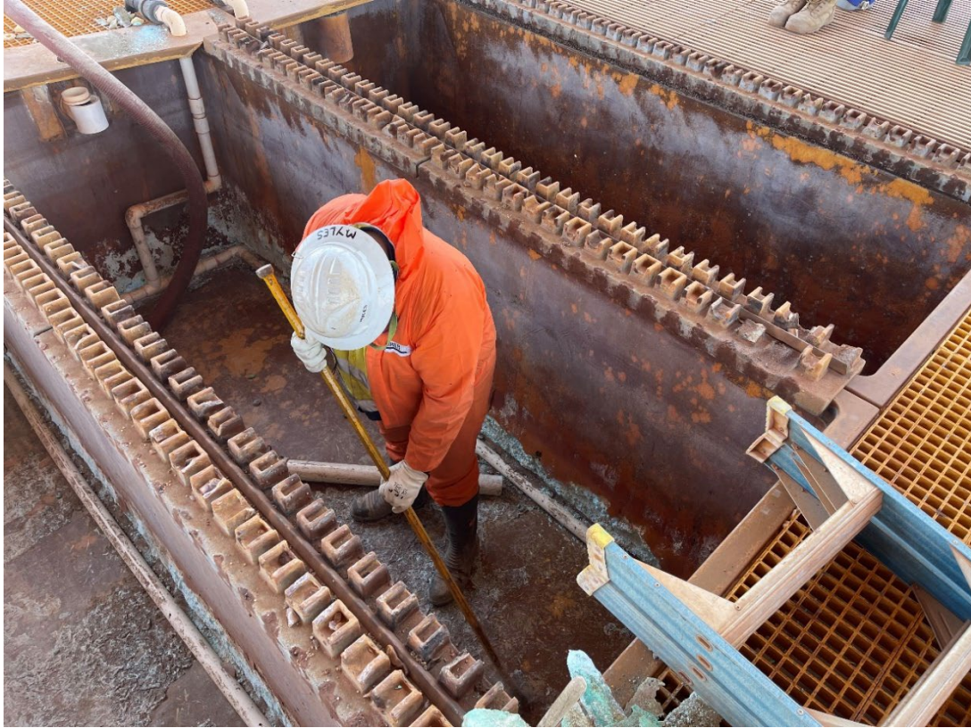
Image 8 / Cleaning out EW Cells post Hydro testing
