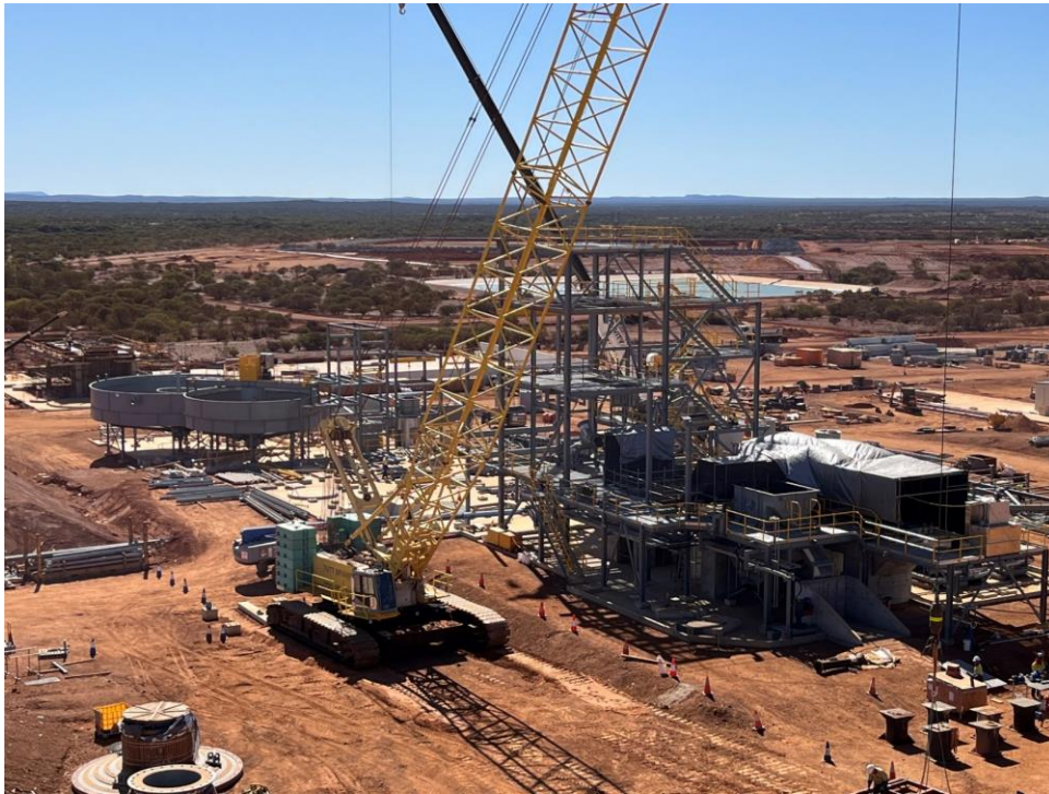
Figure 6. Processing plant construction, mill, flotation, thickening and concentrate sections (July Photo).
