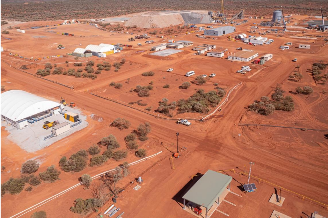
Figure 4. Work progress at the main Abra plant and infrastructure area looking West.
