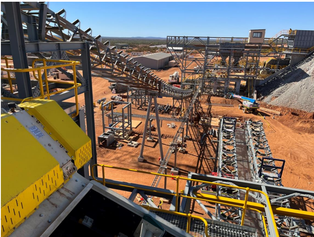
Figure 5. Crusher area with commencement of conveyor installation (July Photo).
