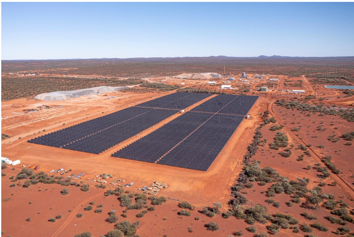
Figure 9. 16,000 solar panels installed in solar farm.
