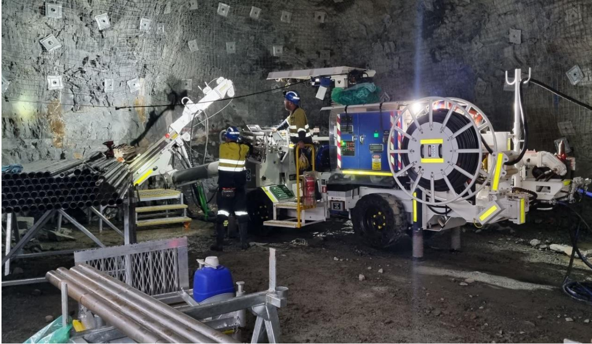
Figure 10. Commencement of underground Drilling at Abra (Swick Mining Services).
