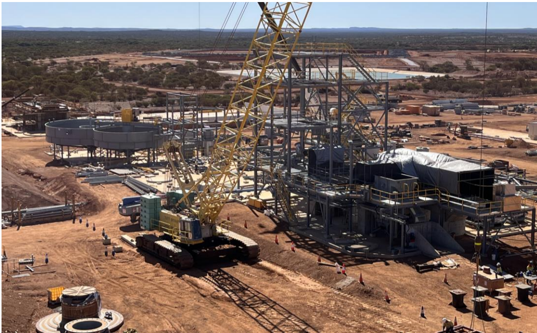
Figure 6: Photo showing construction progress milling, flotation, thickening and filtration circuits (July 2022).
