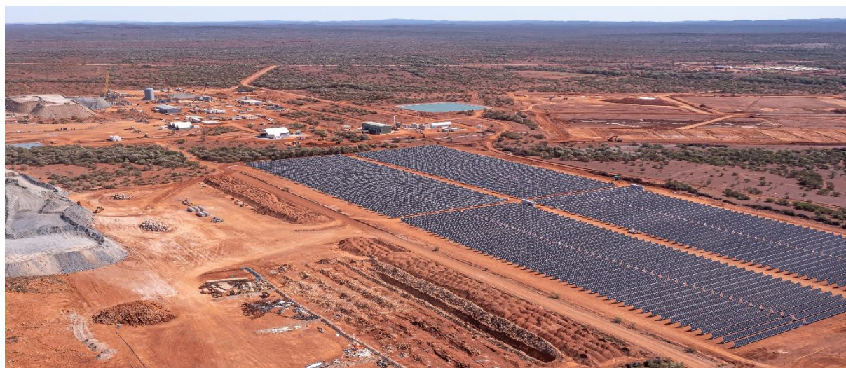
Figure 1 - Abra site with solar farm and village in background (looking west).
