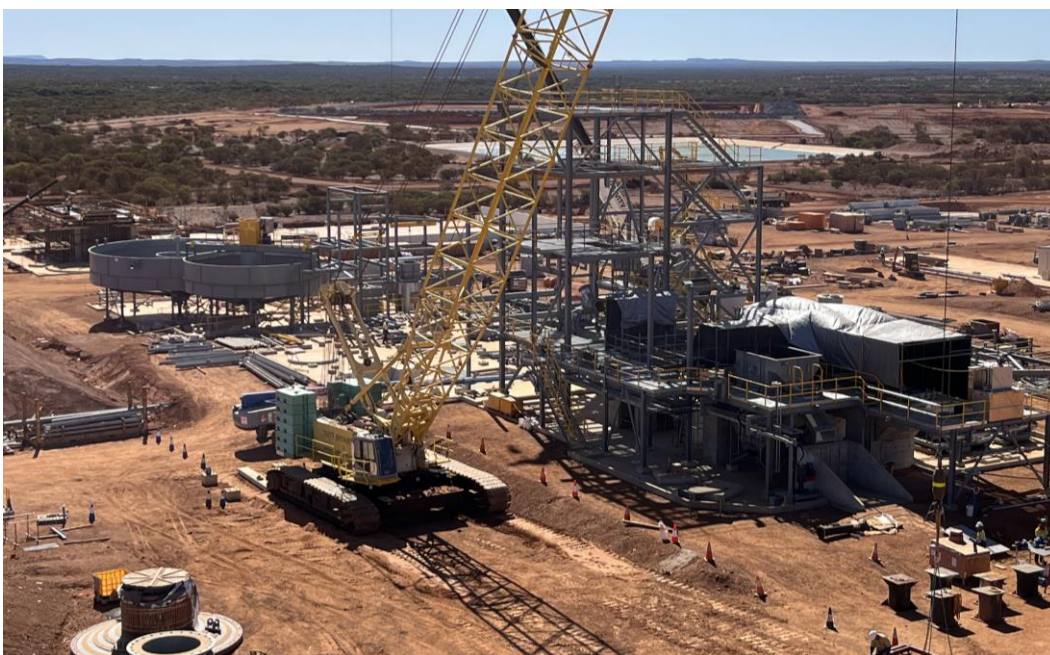
Figure 6: Photo showing construction progress milling, flotation, thickening and filtration circuits (July 2022).
