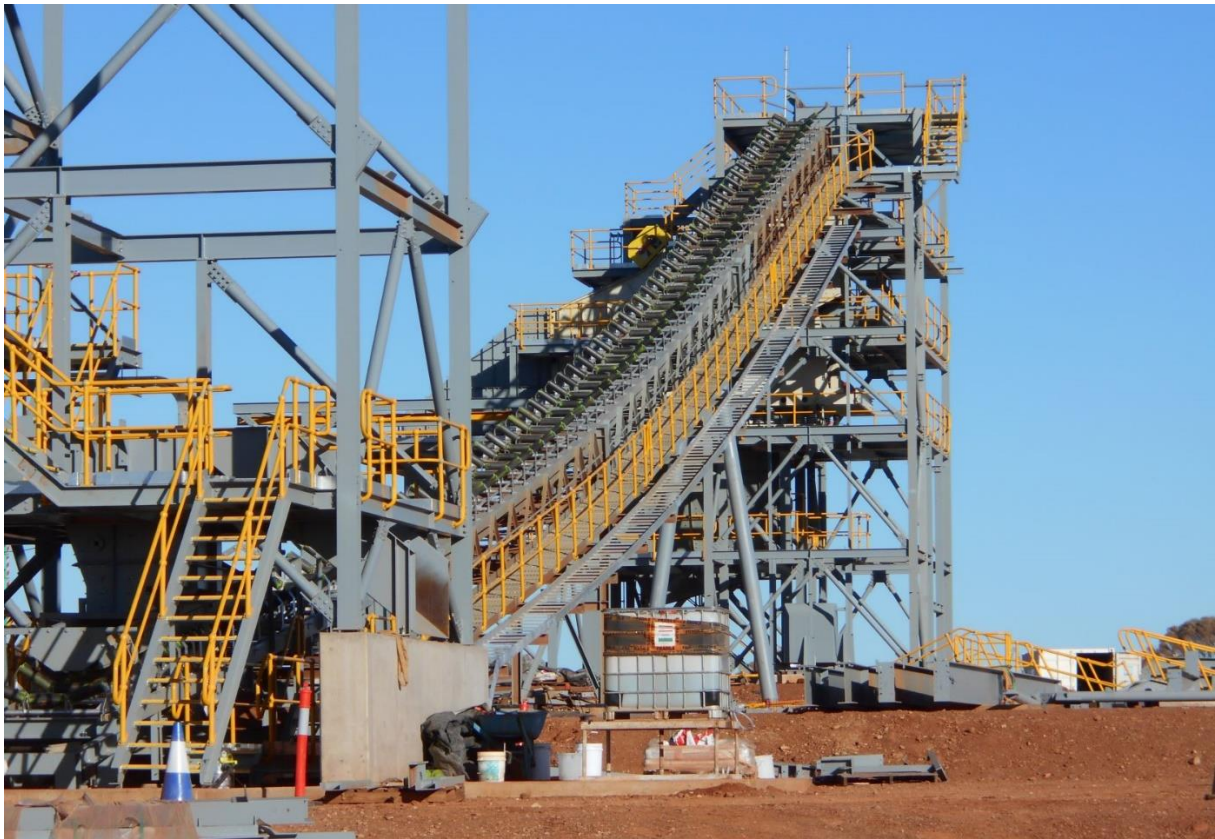
Figure 4 - Abra crushing and screening sections.
