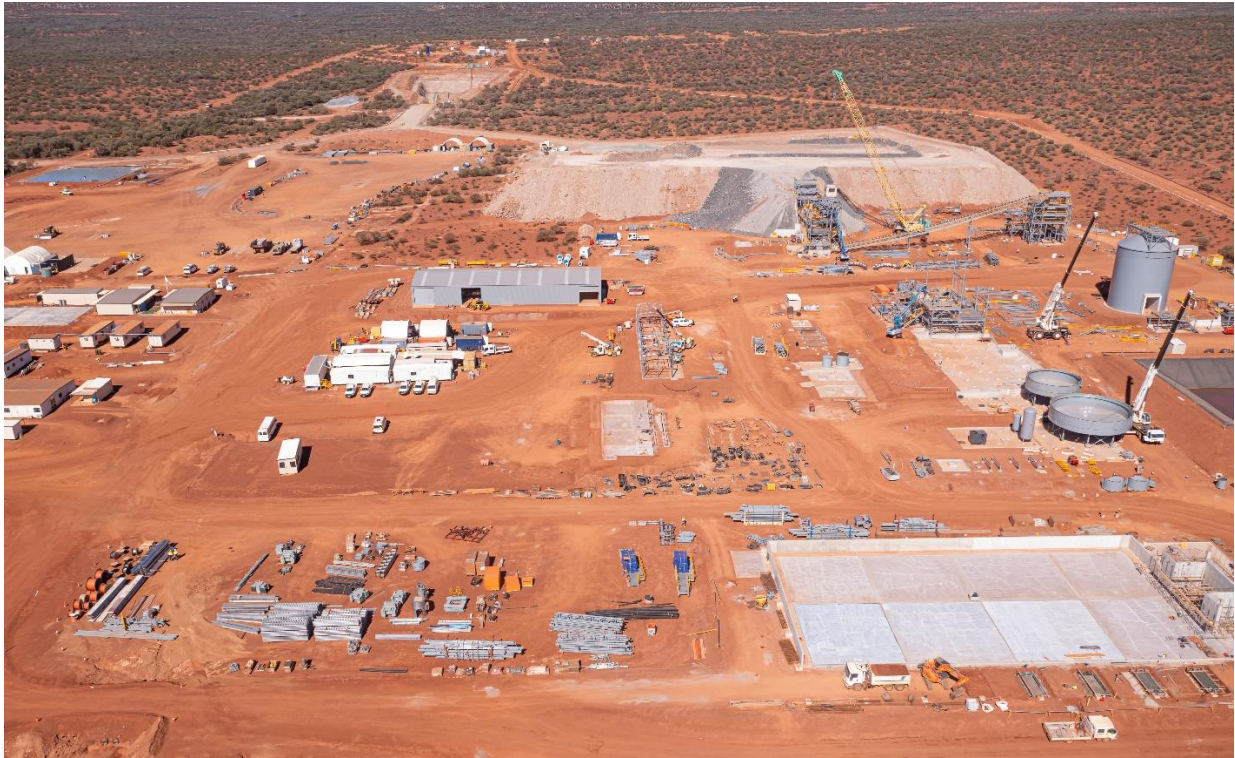
Figure 2 - Abra processing plant construction (looking south).
