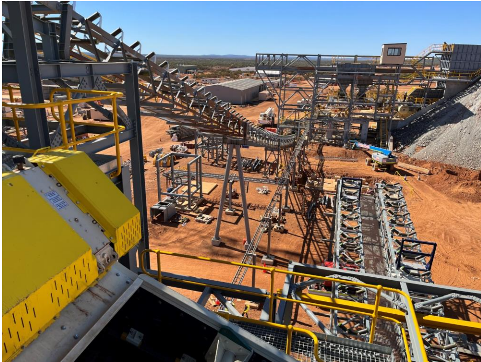
Figure 5 – Abra crushing & Screening sections steel erection (photo: 12 July)
