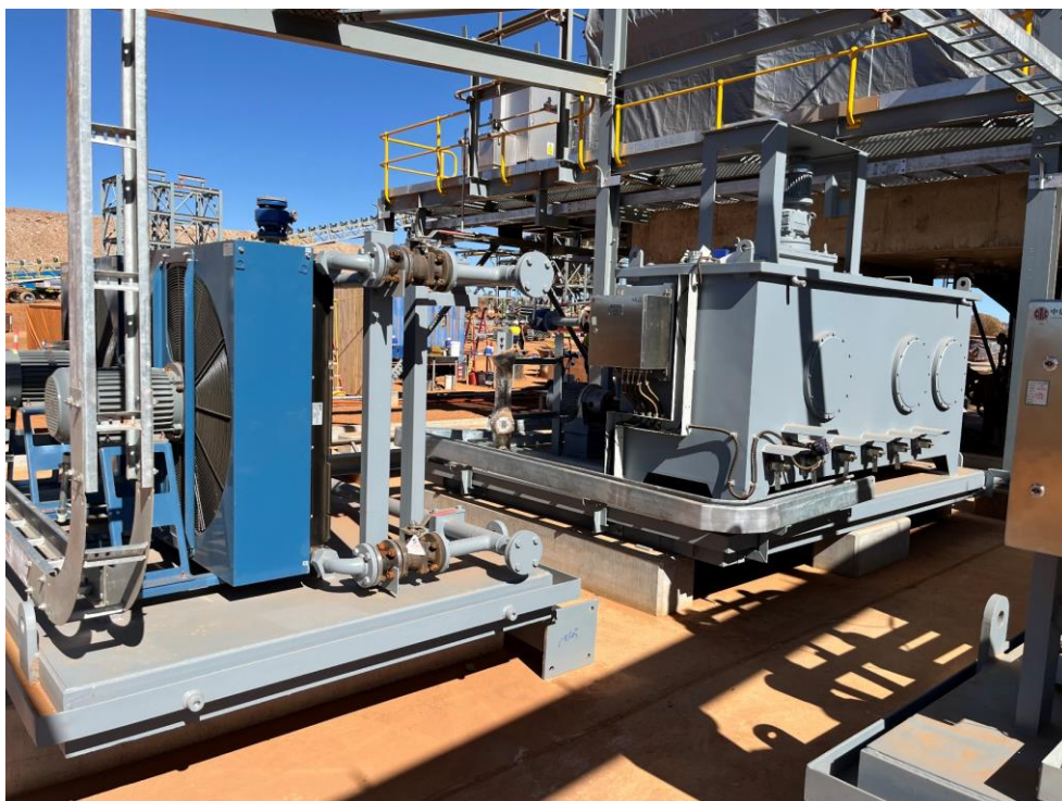
Figure 6 – Mill bearing lubrication equipment (photo: 12 July).
