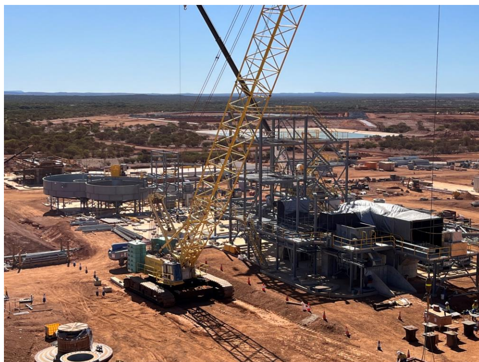
Figure 4 – Processing plant construction, mill, flotation, thickening and concentrate sections (photo: 12 July 2022).
