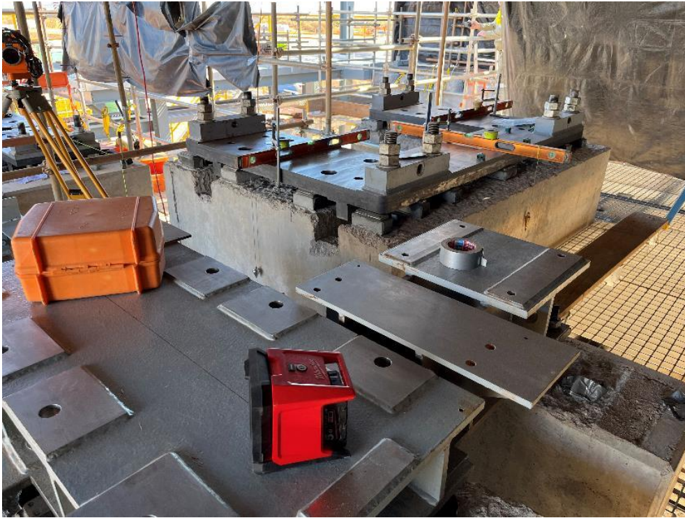
Figure 7 – Mill drive train sole plates (Photo taken 12 July 2022).
