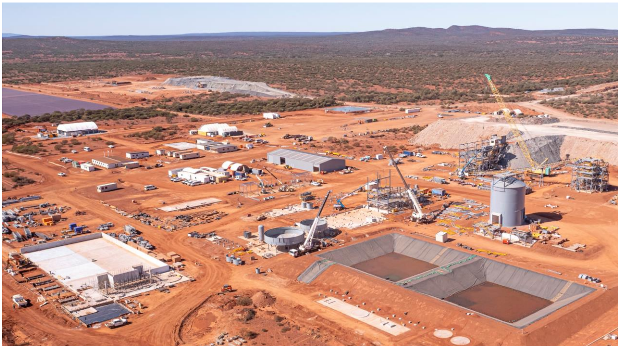
Figure 1 – Abra mine construction site (photo: 28 June 2022)
