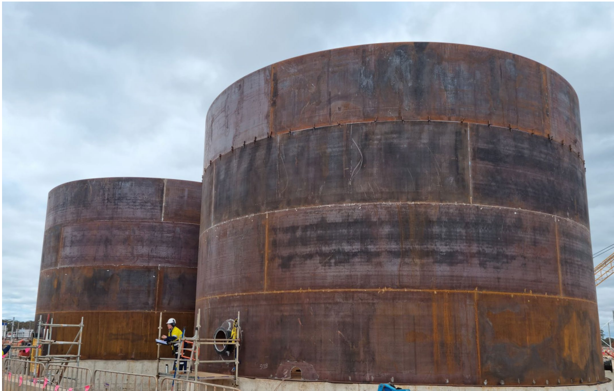
Fabrication of two 1300m 3 tanks complete
