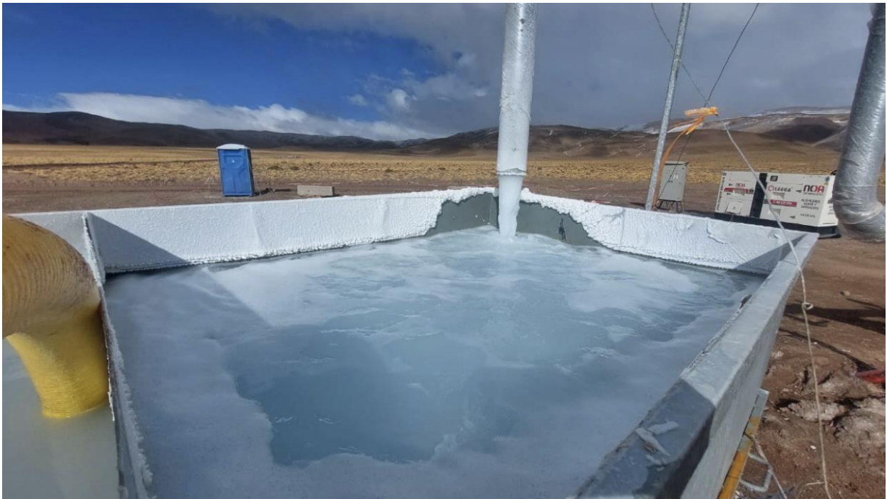
Figure 2 – Brine discharge at PBPP-01-21 during long term pumping test.
