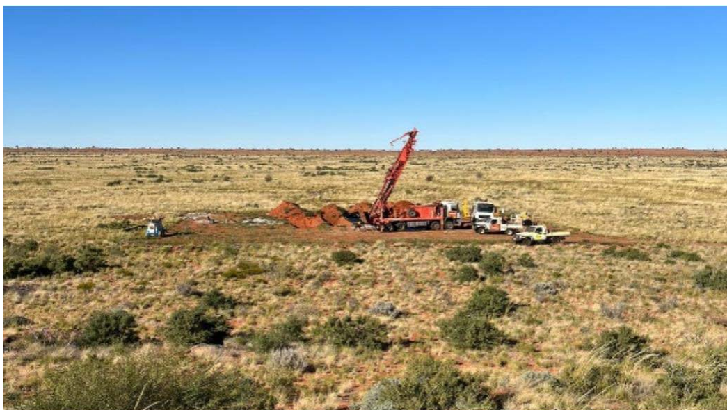
Figure 1: Drill Rig at Paterson Central Project.
