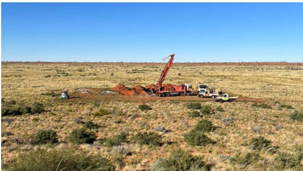
Figure 1: Drill Rig at Paterson Central Project.
