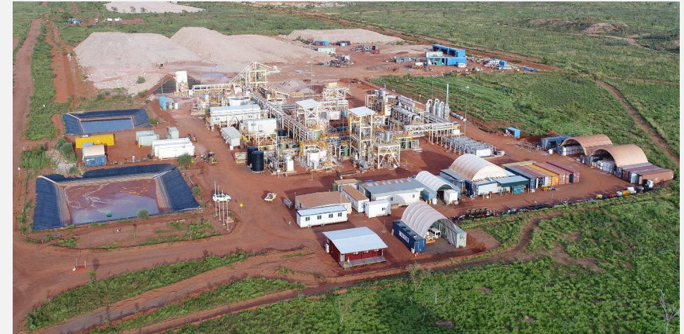
Northern Minerals Limited Browns Range Pilot Plant
