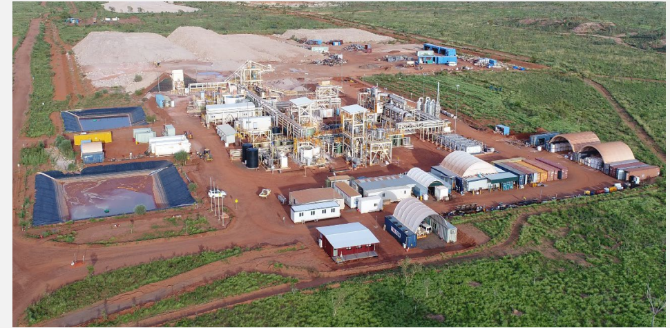
Northern Minerals Limited Browns Range Pilot Plant
