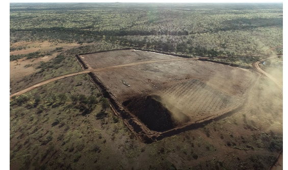
Figure 6. First blast successfully completed and ready for excavation.
