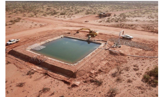
Figure 4. Turkeys nest for construction water
