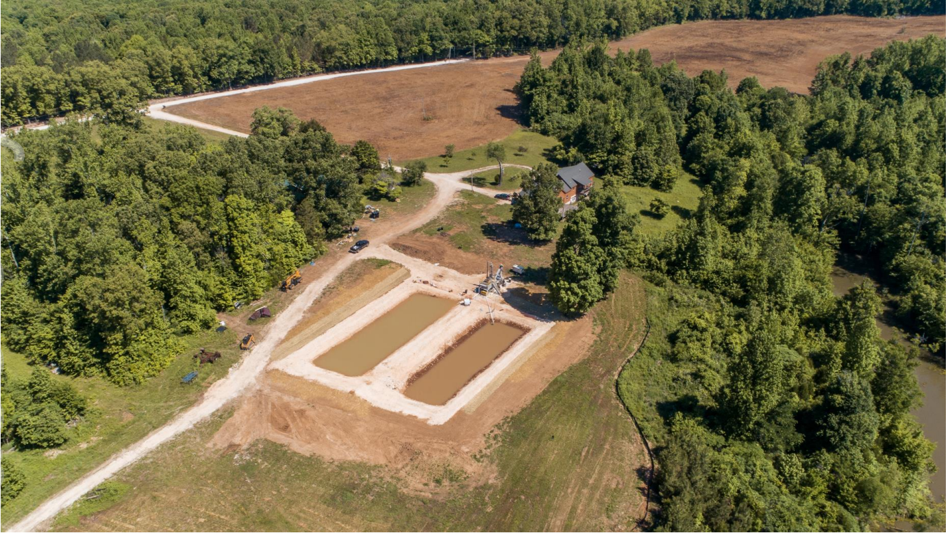
Figure 12: Titan Project Mineral Demonstration Facility.
