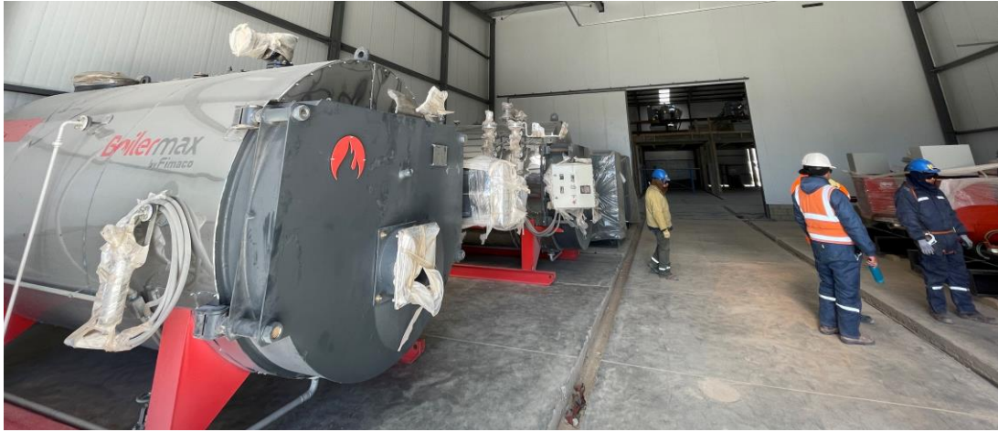
Figure 2. Rincon Lithium Project – 2,000tpa Operation Site Works
