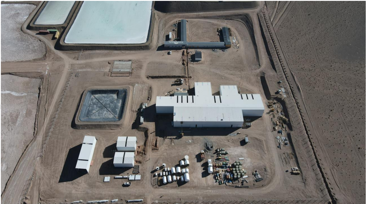
Figure 1. Rincon Lithium Project – 2,000tpa Operation Site Works
