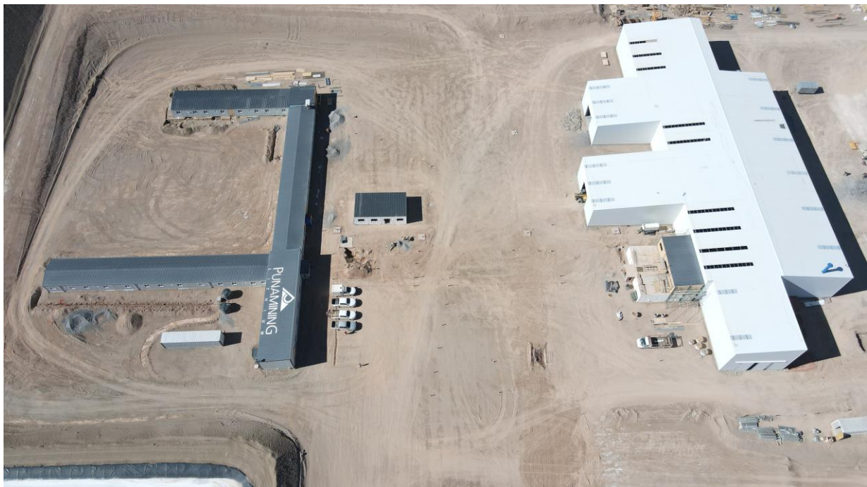
Figure 4. Rincon Lithium Project – 2,000tpa Operation Site Works
