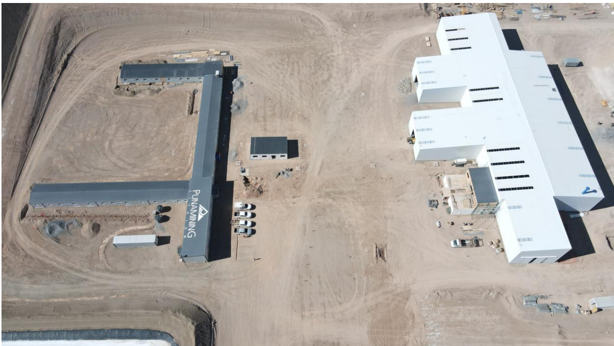
Figure 4. Rincon Lithium Project – 2,000tpa Operation Site Works
