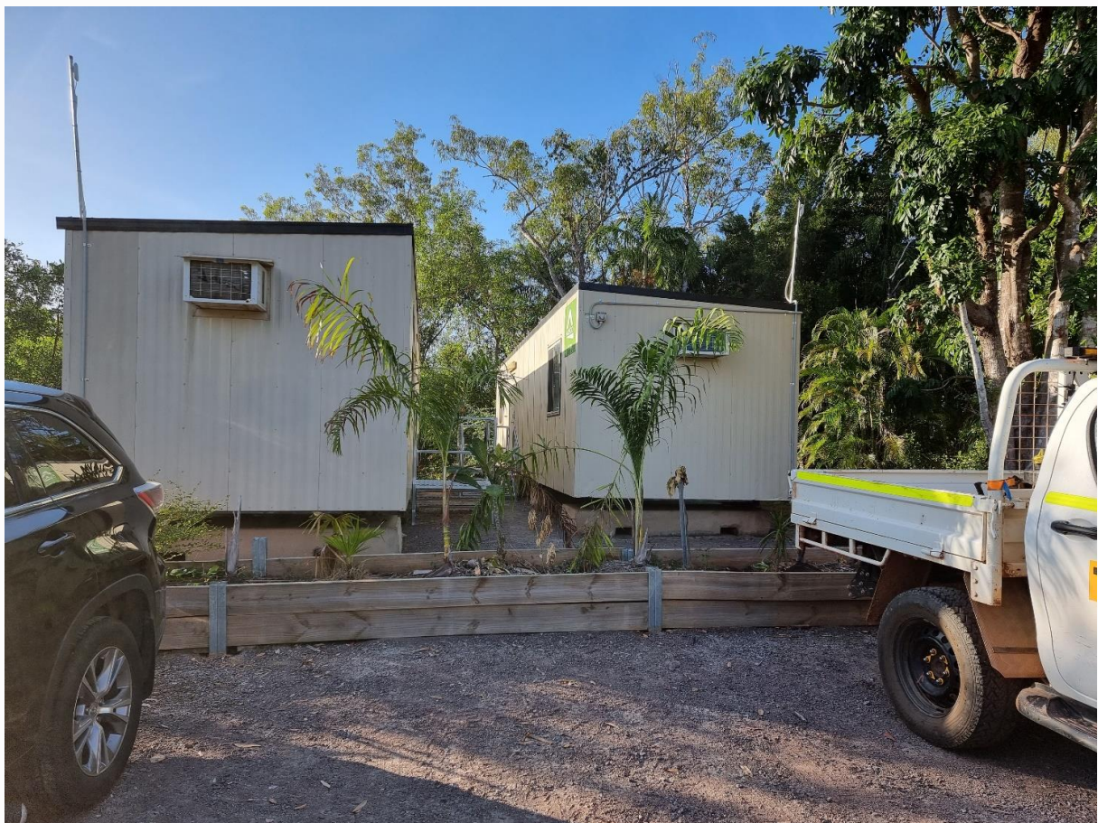
Figure 4.. Tumbling waters temporary administration building
