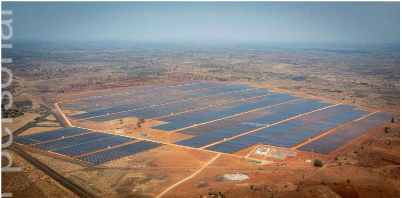
Figure 28: 60MW Salima Solar Power Plant in Malawi recently constructed and commissioned by JCM (source: JCM)
