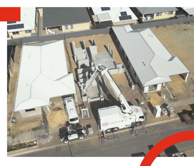
Can lay multiple types of existing blocks from multiple block manufacturers
