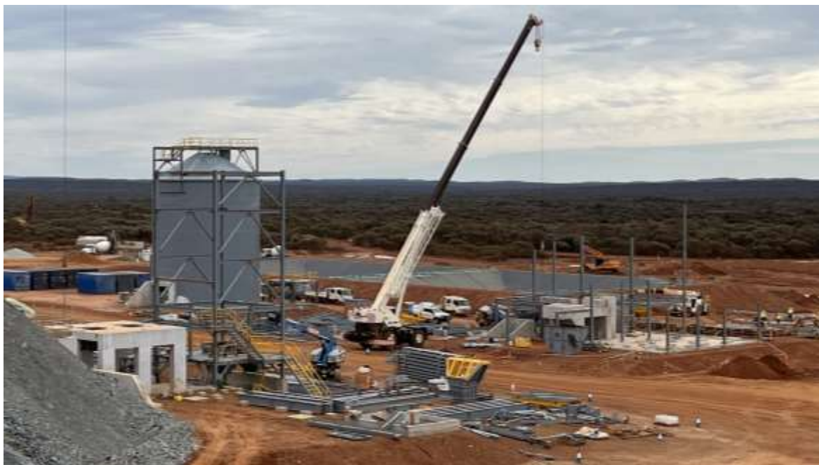
Figure 1 shows the Abra processing plant construction activities in May 2022. Commencement of structural steel installation for the crusher and mill areas in front of the completed fine ore bin (FOB).
