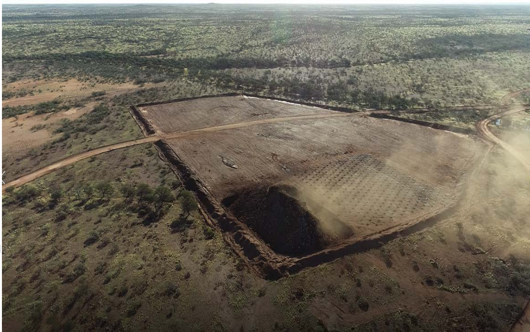
Figure 2. First blast successfully completed and ready for excavation.
