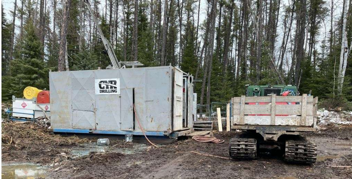
Figure 11: Drill rig set up on hole MF22-77
