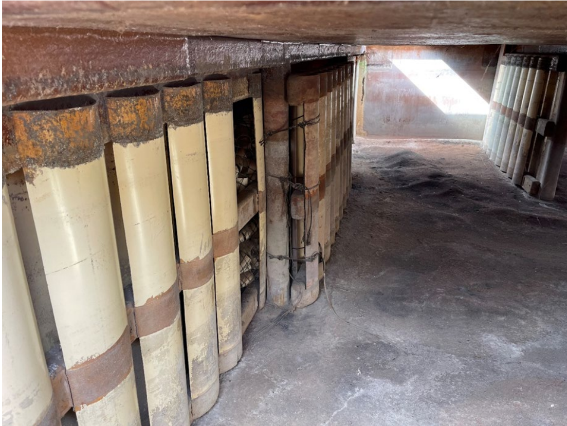
Image 4 / SX Mixer Settler cleanout lower level – after
