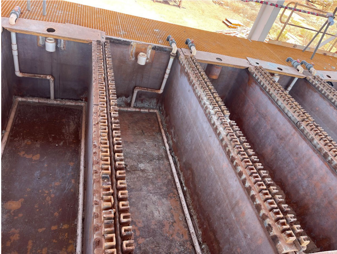
Image 8 / Cleaned EW Cells ready for condition inspection
