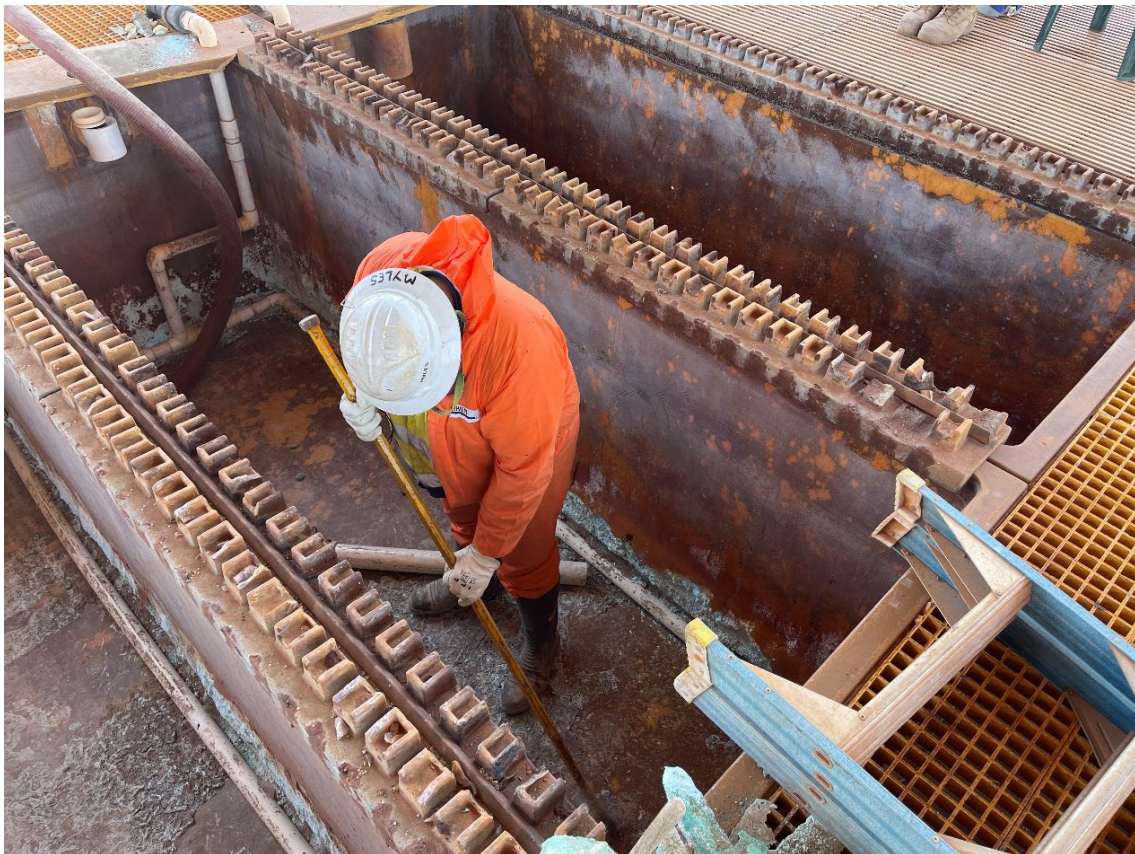
Image 7 / Cleaning out EW Cells post Hydro testing
