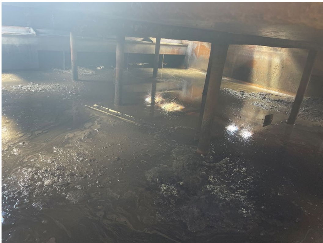
Image 3 / SX Mixer Settler cleanout lower level – before
