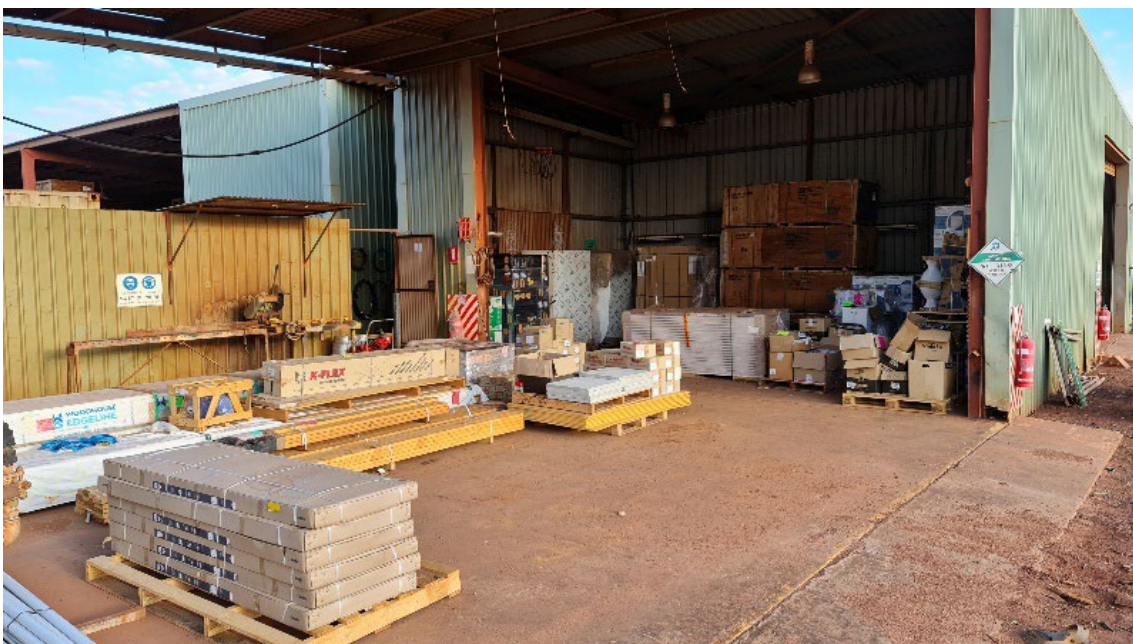
Image 9 / Accommodation Refurbishment Materials
