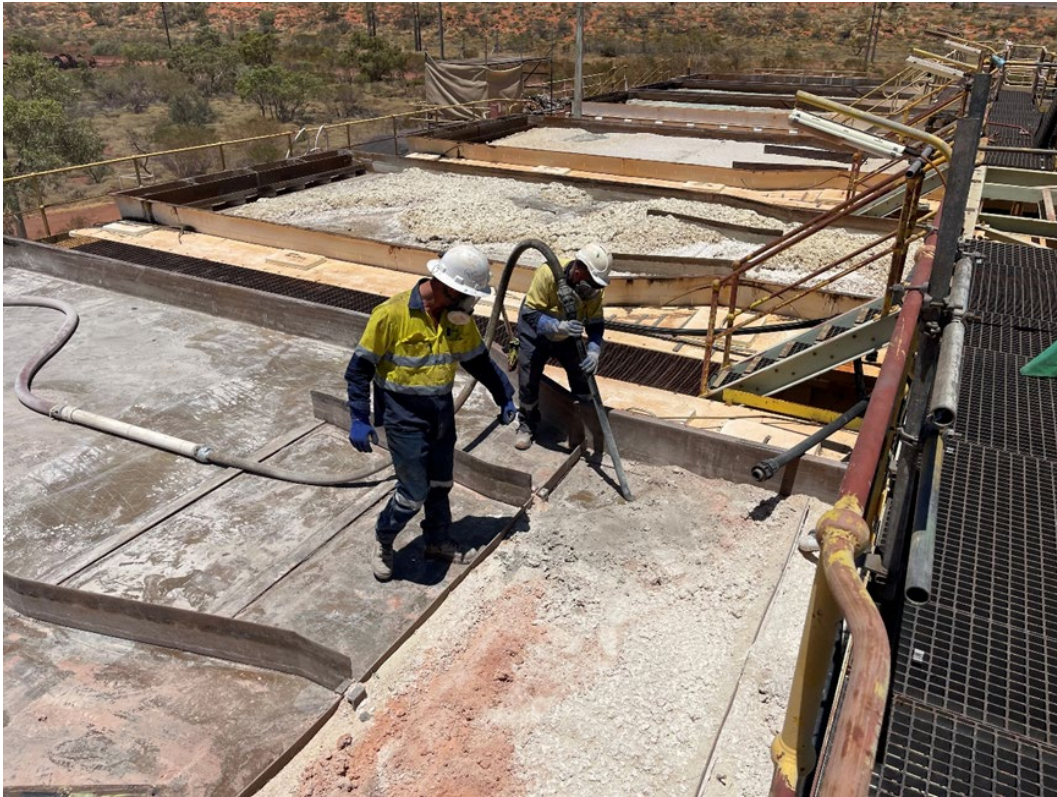
Image 2 / SX Mixer Settler clean-up top level
