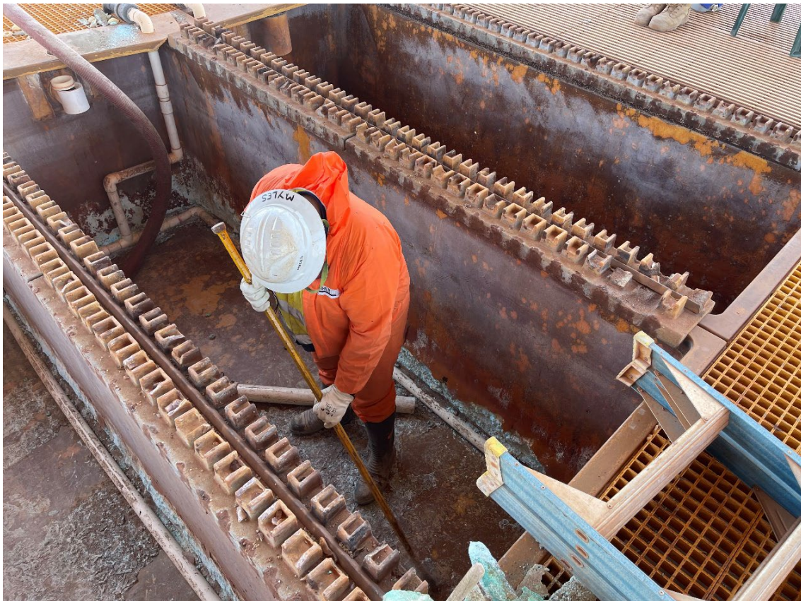
Image 7 / Cleaning out EW Cells post Hydro testing
