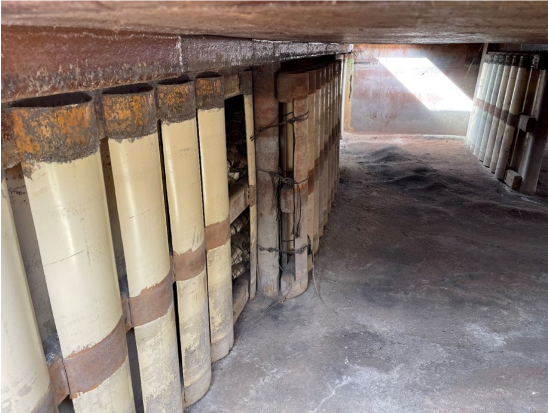
Image 4 / SX Mixer Settler cleanout lower level – after
