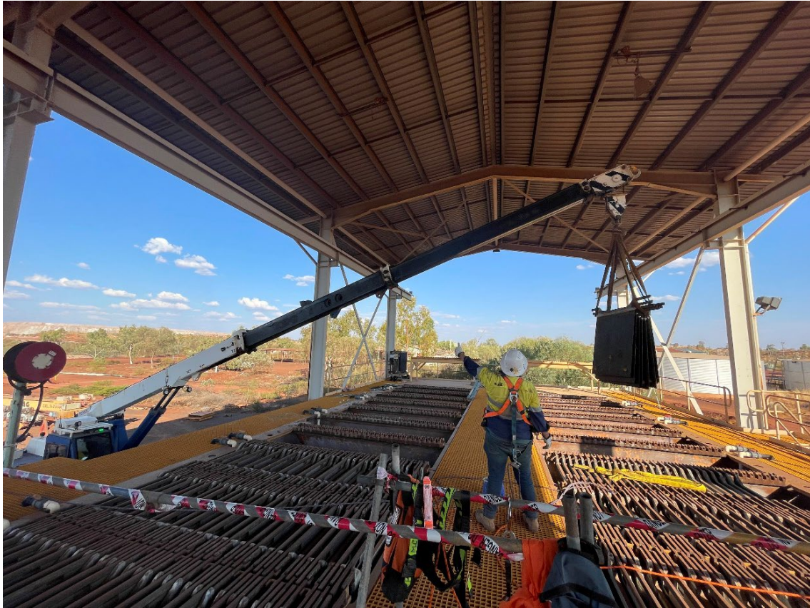
Image 6 / EW - Anode removal
