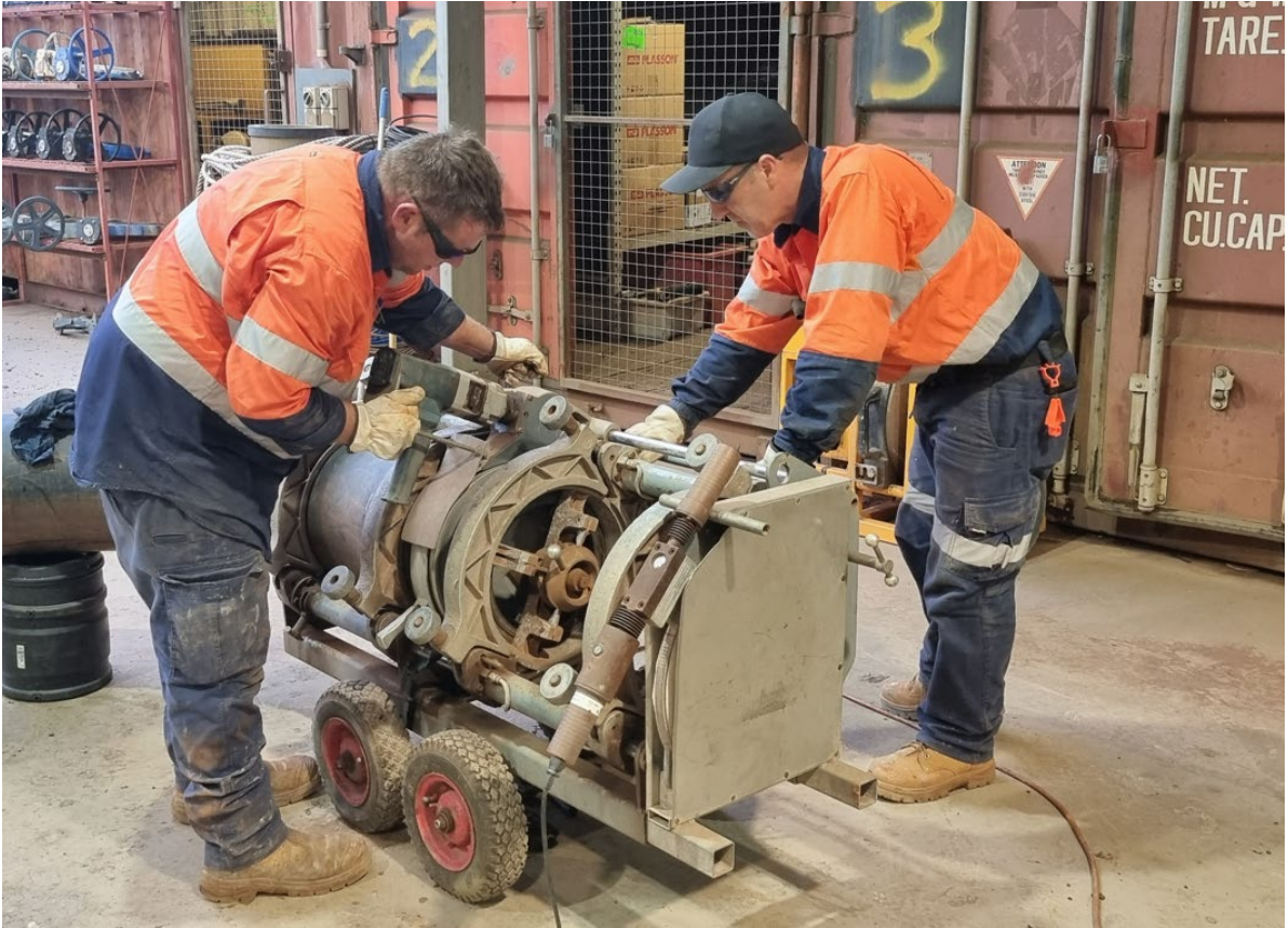
Image 14 / Repairing of piping and equipment
