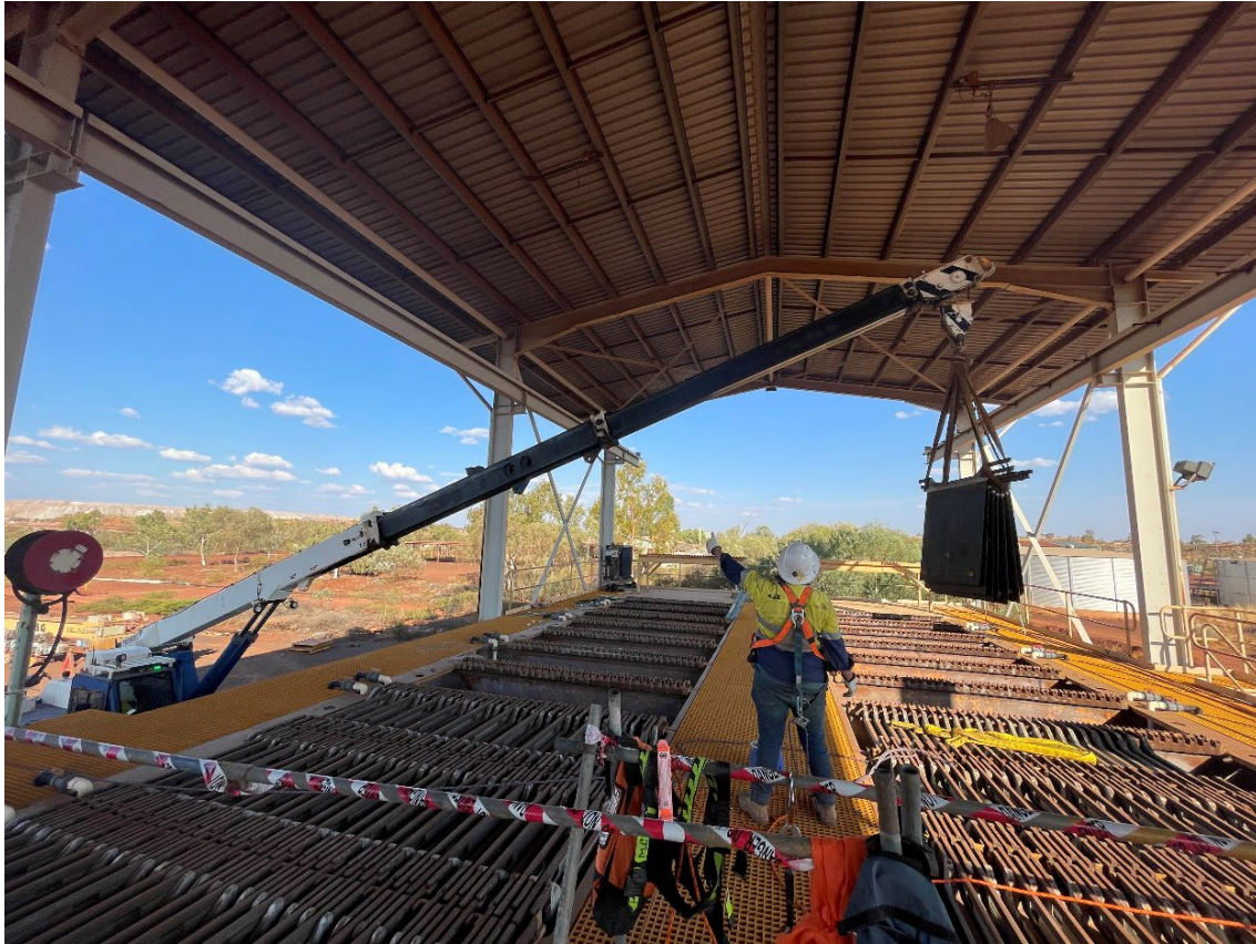
Image 6 / EW - Anode removal
