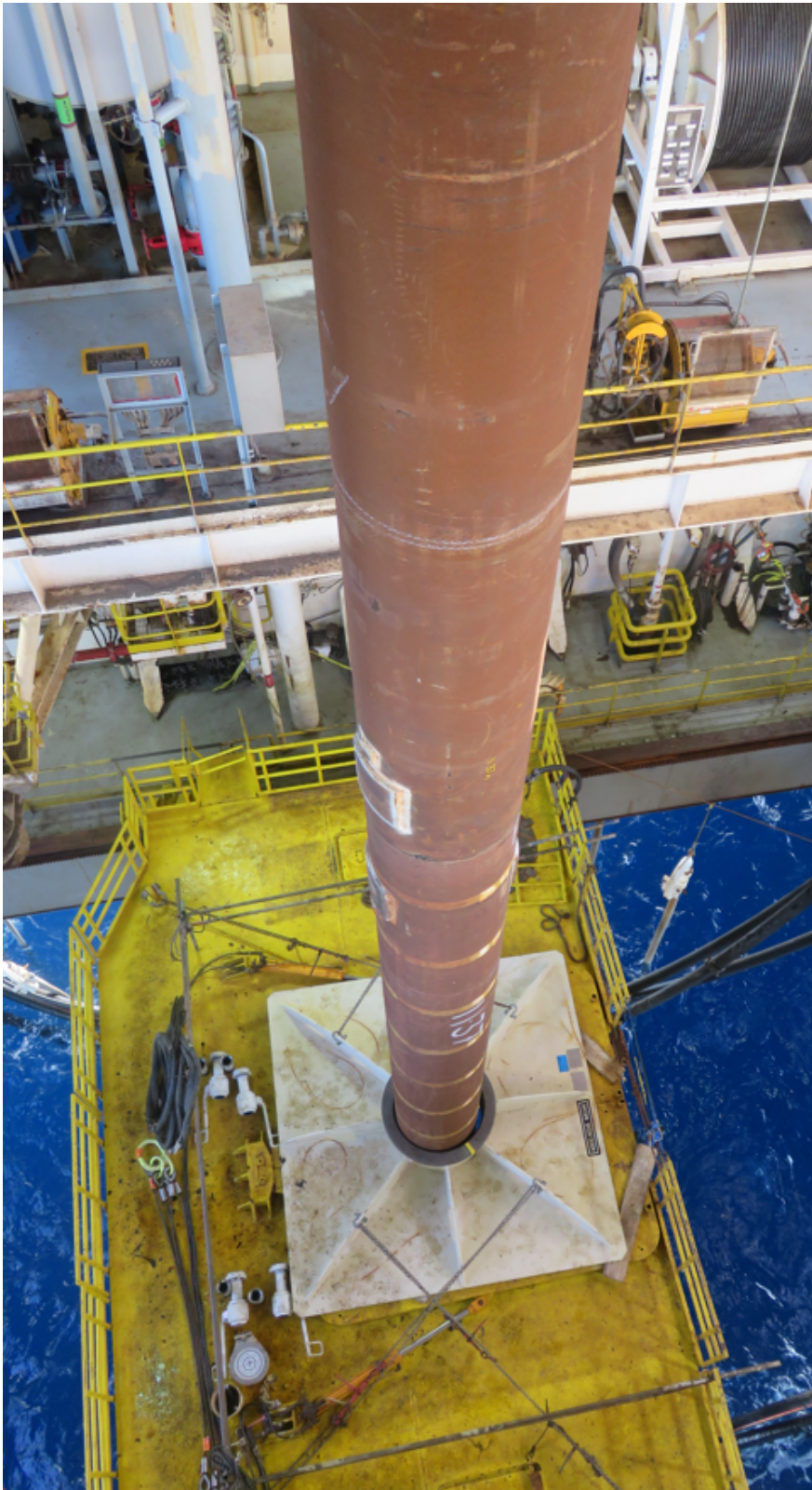
36" Conductor and mudmat being made up prior to deployment.
