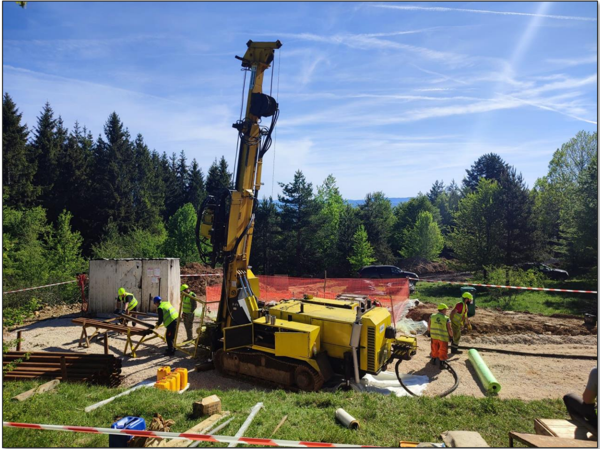
Figure 1: Drilling rig at the RDK prospect, May 2022
