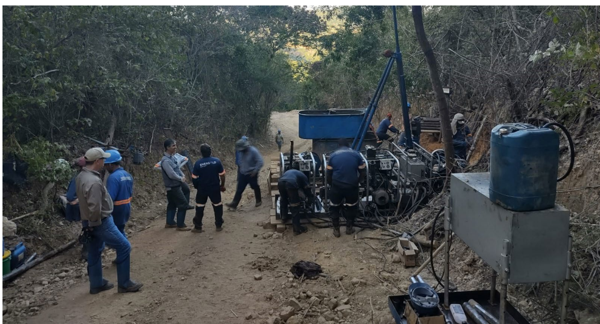
Figure 6: Establishment and drill-rig set-up of drillhole MADD003, Monte Alto Prospect – Salinas Lithium Project, Brazil
