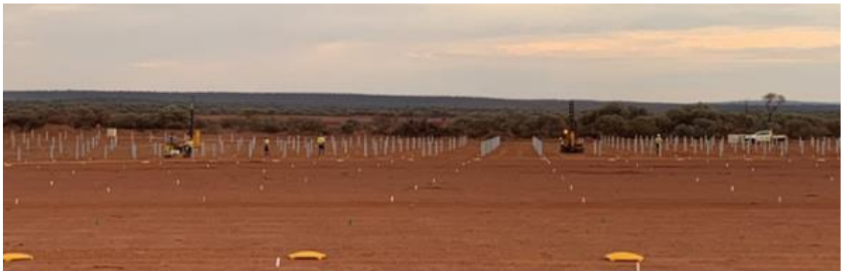
Figure 13 – Post-hole drilling and piling prior to commencement of solar panel installation.
