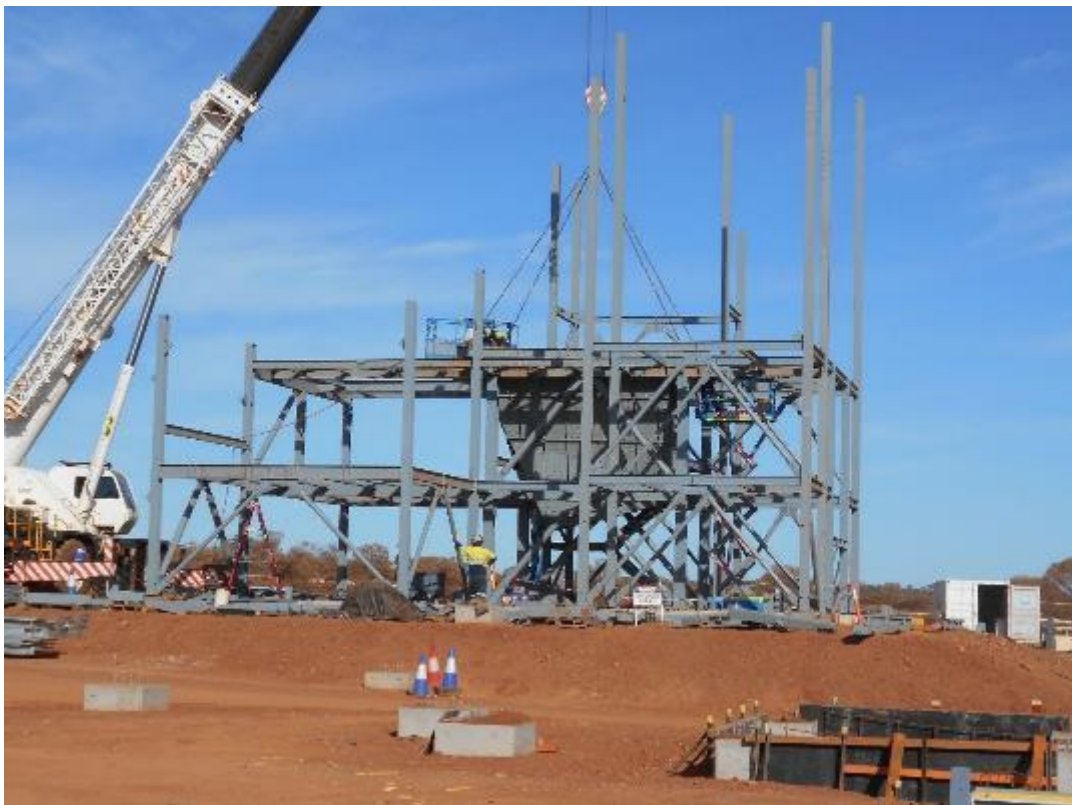
Figure 7 – Crushing screening area steelwork.
