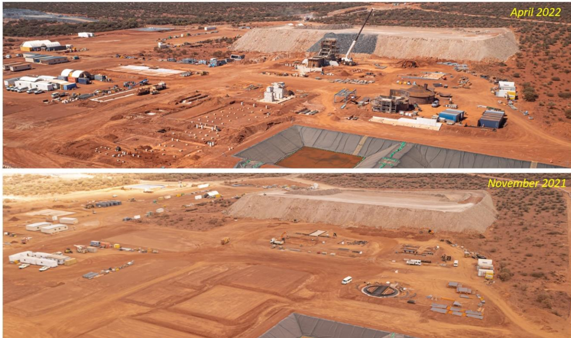
Figure 2 – Shows work progress on site from November 2021 through to April 2022.
