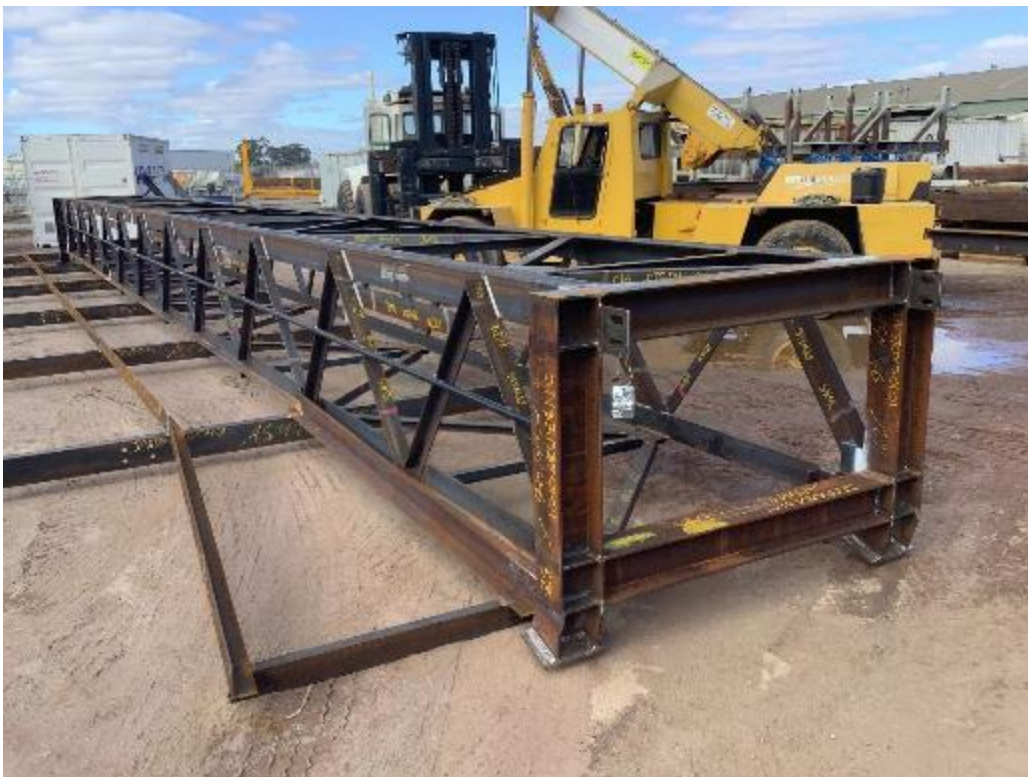
Figure 9 – Conveyor truss fabrication in Perth.
