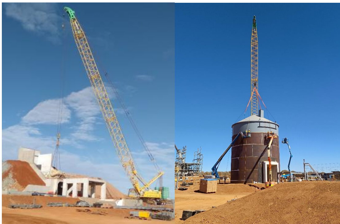
Figure 1 – Lifting of the primary jaw crusher and fine ore bin top into position.
