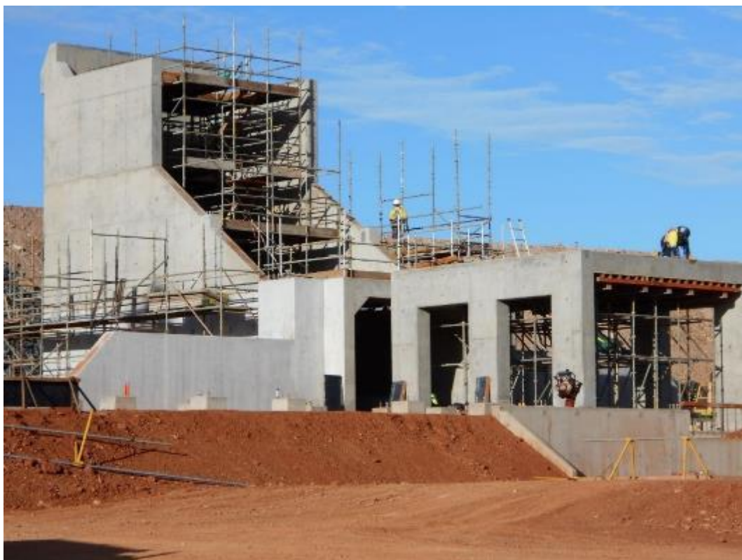
Figure 5 – Crusher concrete complete.
