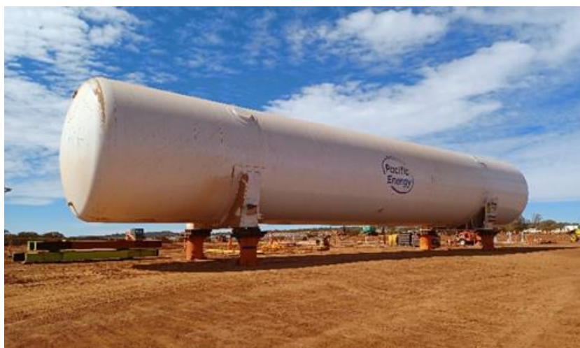
Figure 14 – Arrival on site of first LNG tank (10 May 2022).
