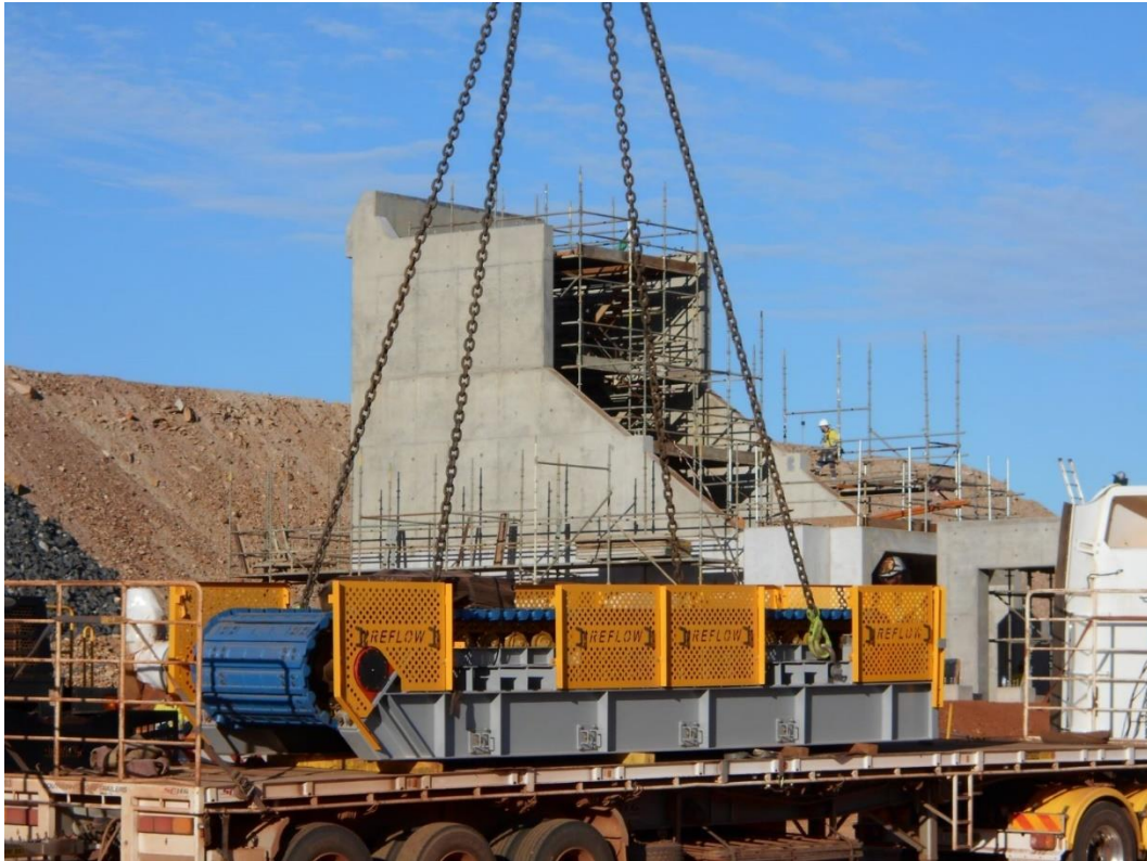
Figure 6 – Arrival of primary crusher feeder.
