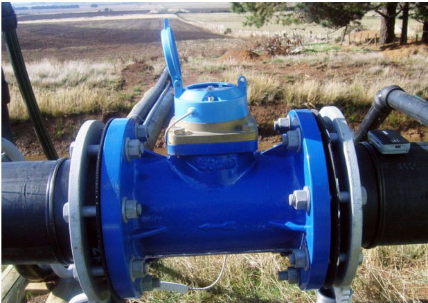
^Photo: Water Meter Used to prevent theft of water Often utilises tamper proof technology
