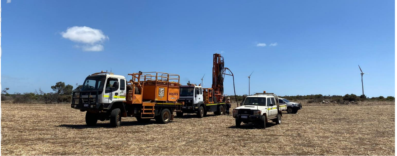
Figure 4: Bostech drilling rig on site
