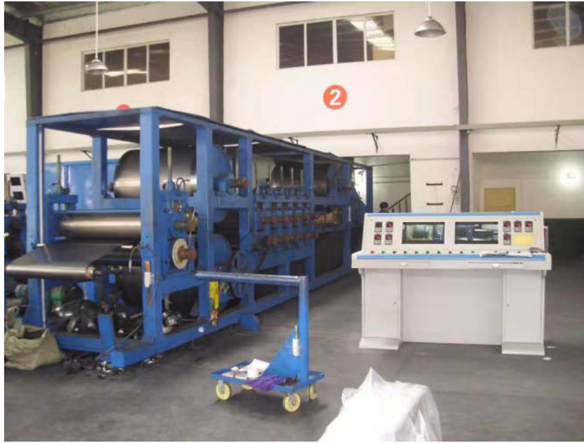
Figure 1: Graphite foil production line at YXGC's Yichang plant
