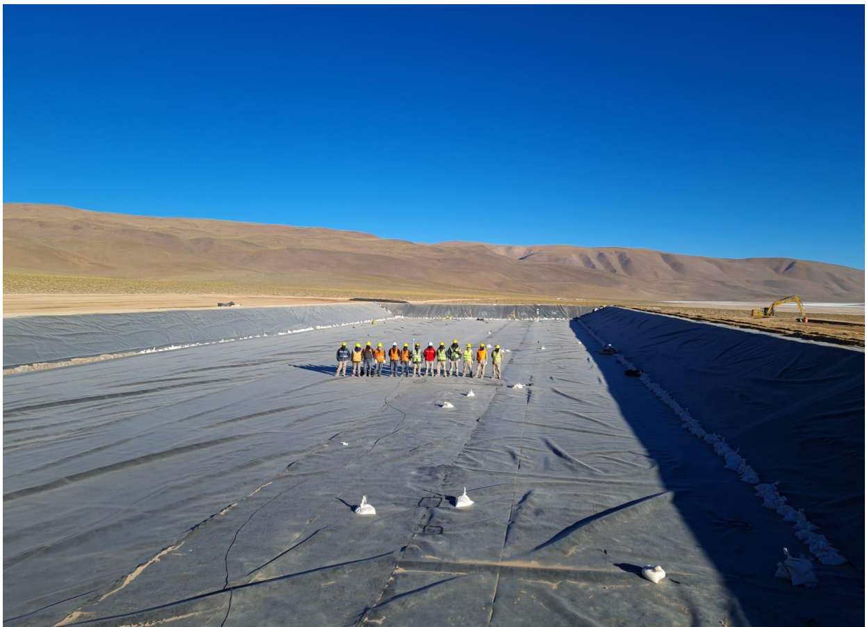
Figure 3: Evaporation Pond S1 Construction
