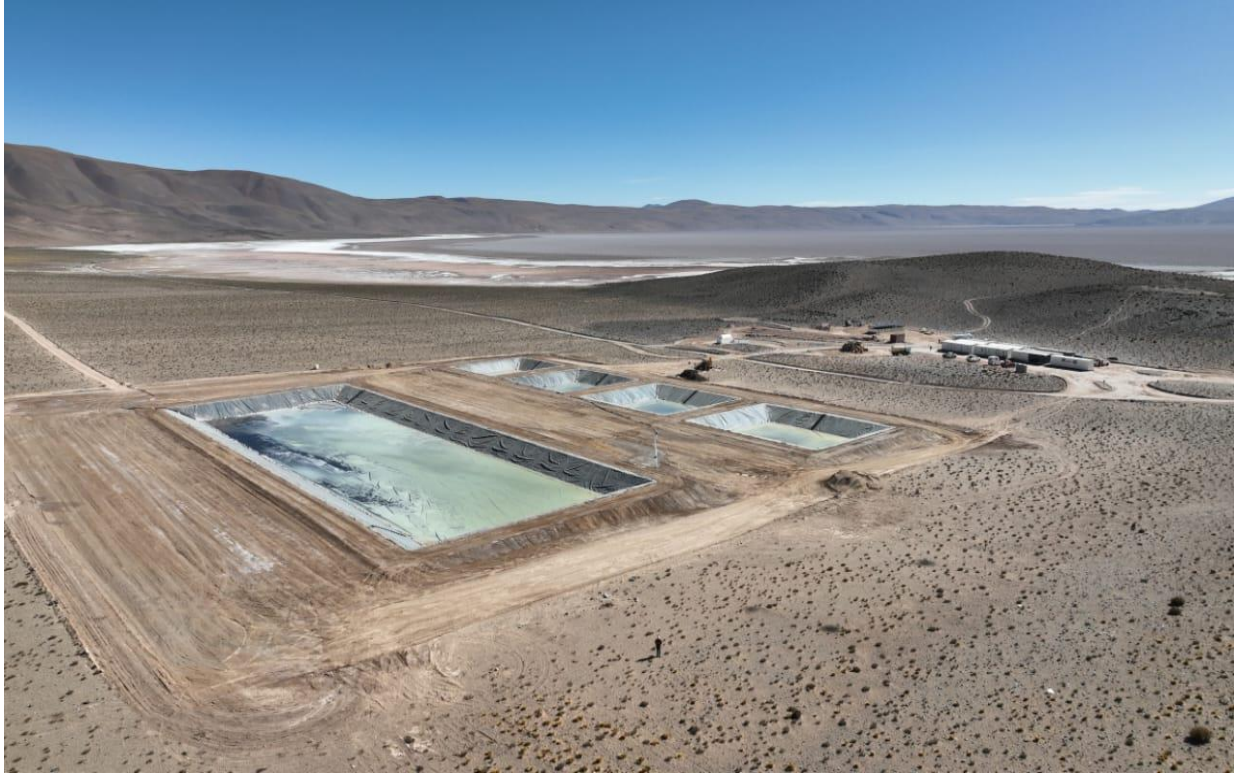
Figure 4: Aerial view of S1 pond filling with brine with camp and the Hombre Muerto salt flat in the background
