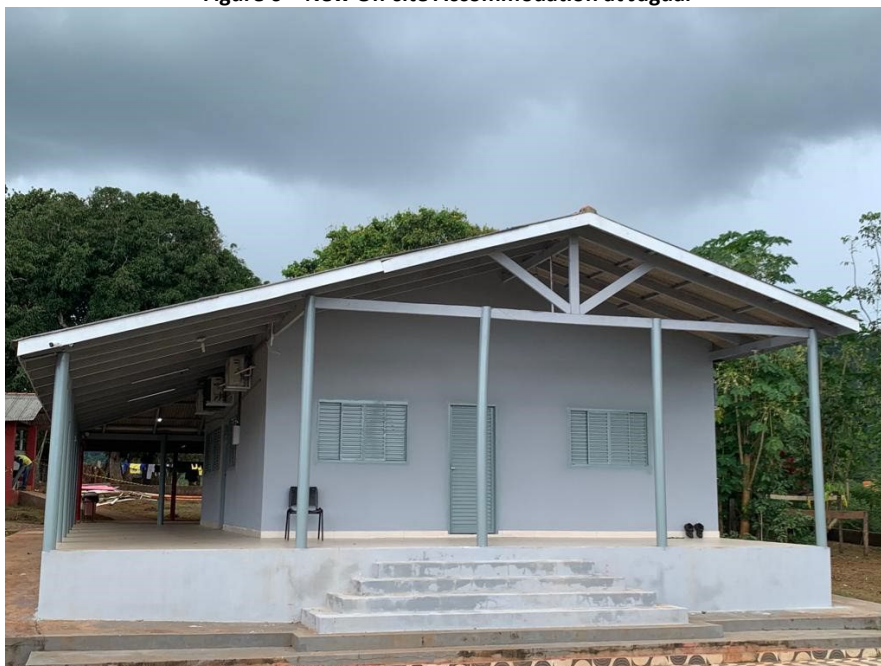
Figure 6 – New On-site Accommodation at Jaguar
