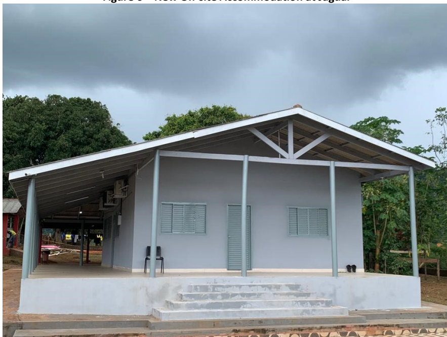
Figure 6 – New On-site Accommodation at Jaguar
